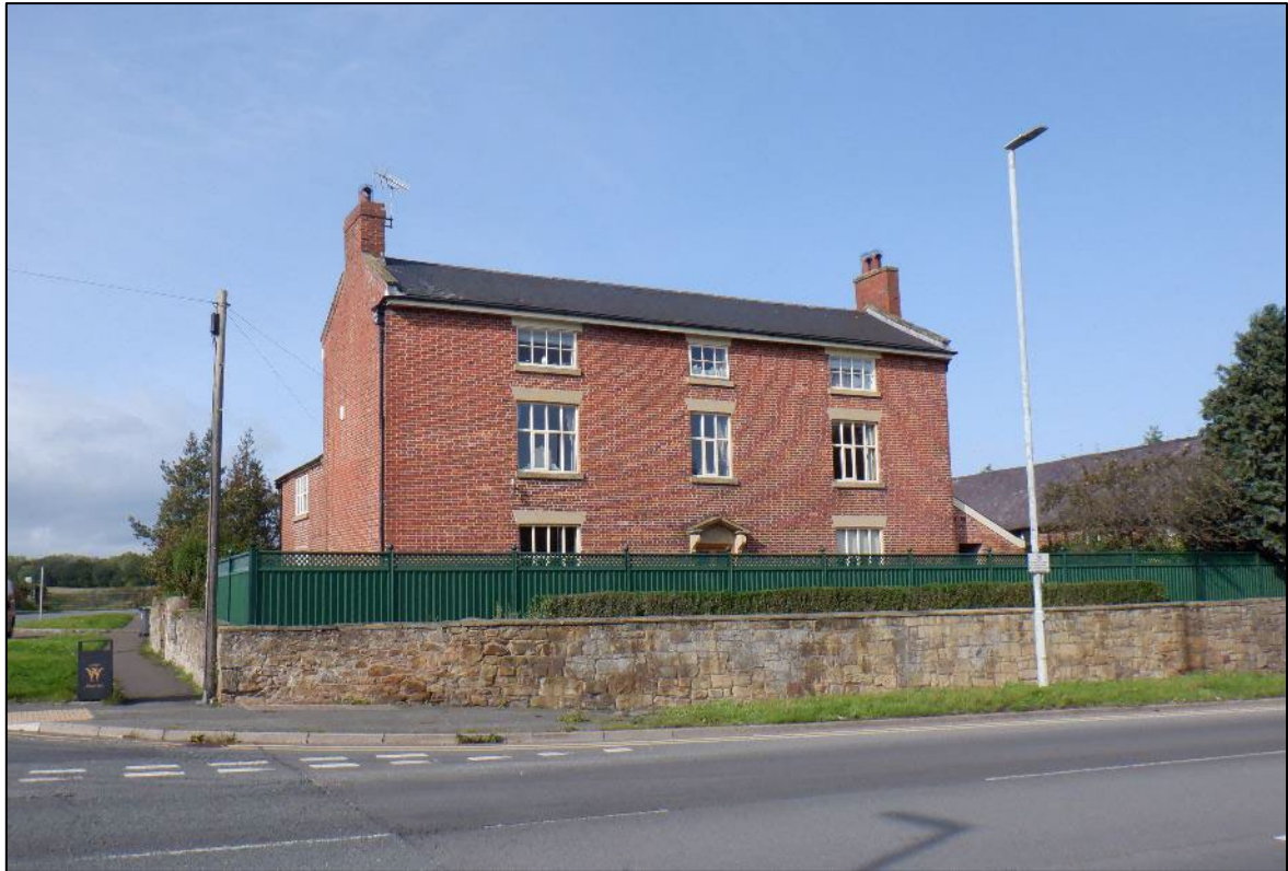
Plate 3. Croesfoel Farmhouse, LB16571, looking north-east.
