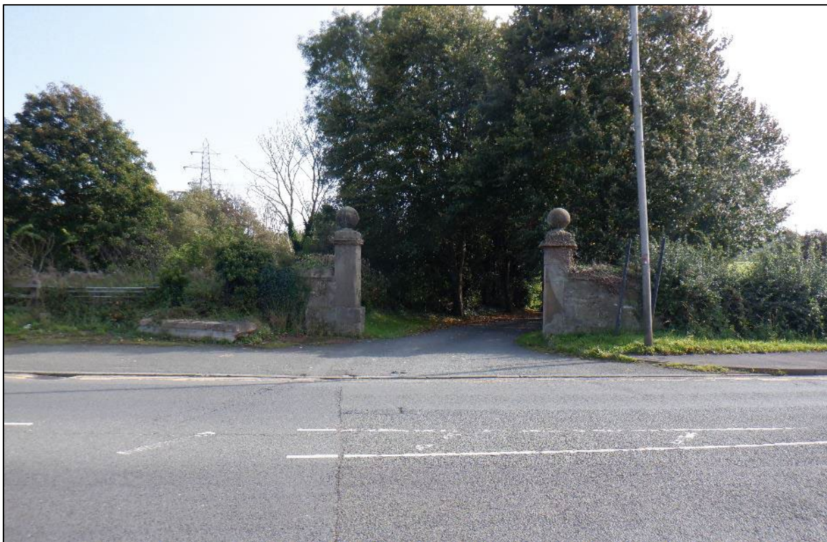
Plate 7. Gate piers at Hafod-y-Bwch, LB16572, looking south.
