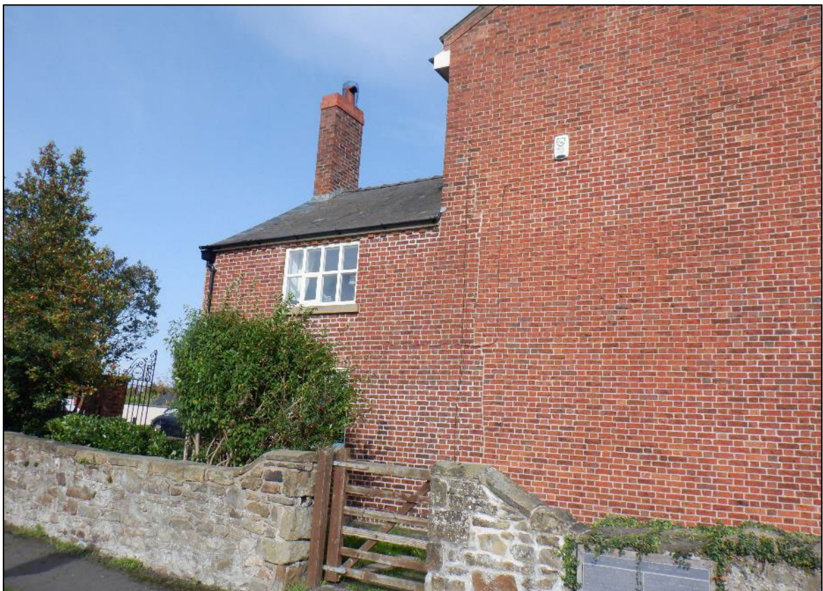
Plate 4. West-facing elevation of Croesfoel Farmhouse, showing side of cross-gable addition to the left, view north-east.
