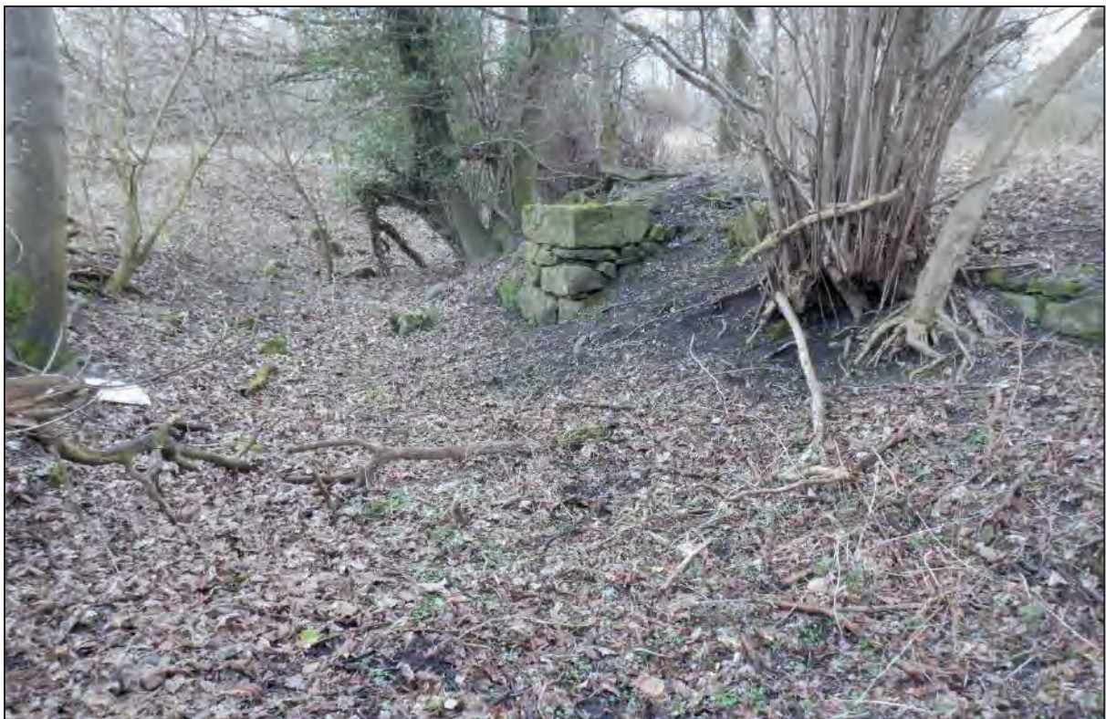
Plate 20. Bridge abutment at Croes-foel moated site, looking north.
