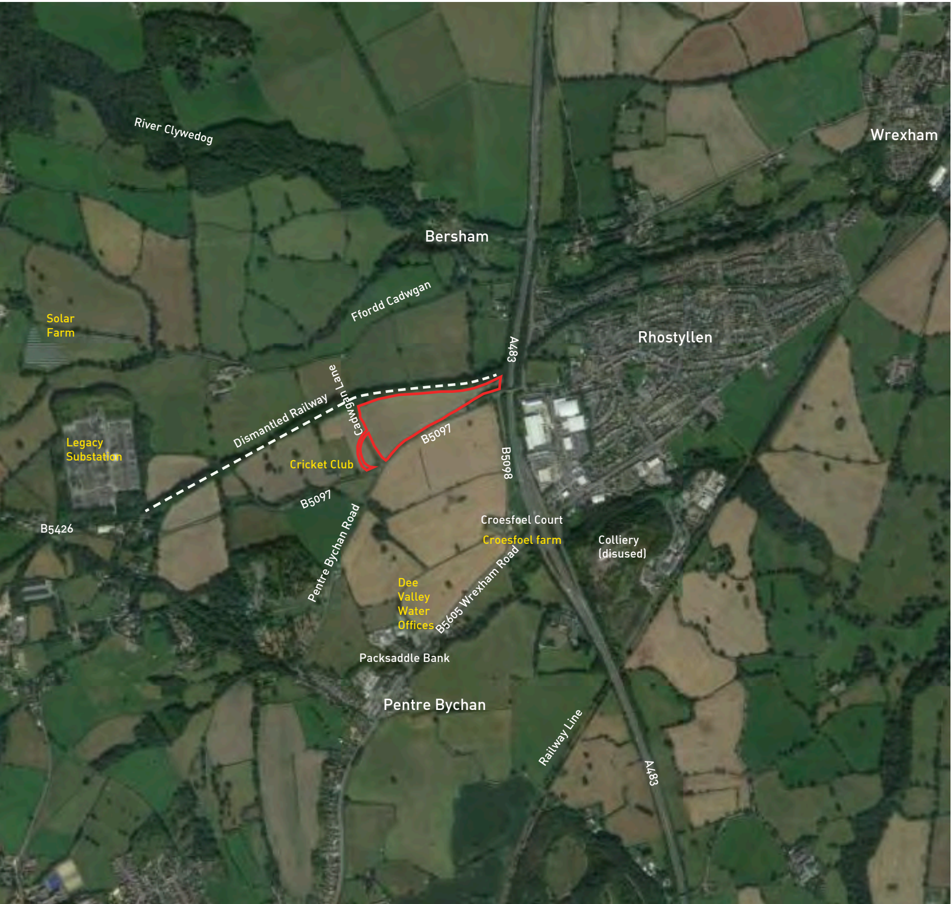
Figure 10. Aerial photography of the site and its surroundings, including red line boundary defining the main development area and access road in the site.
