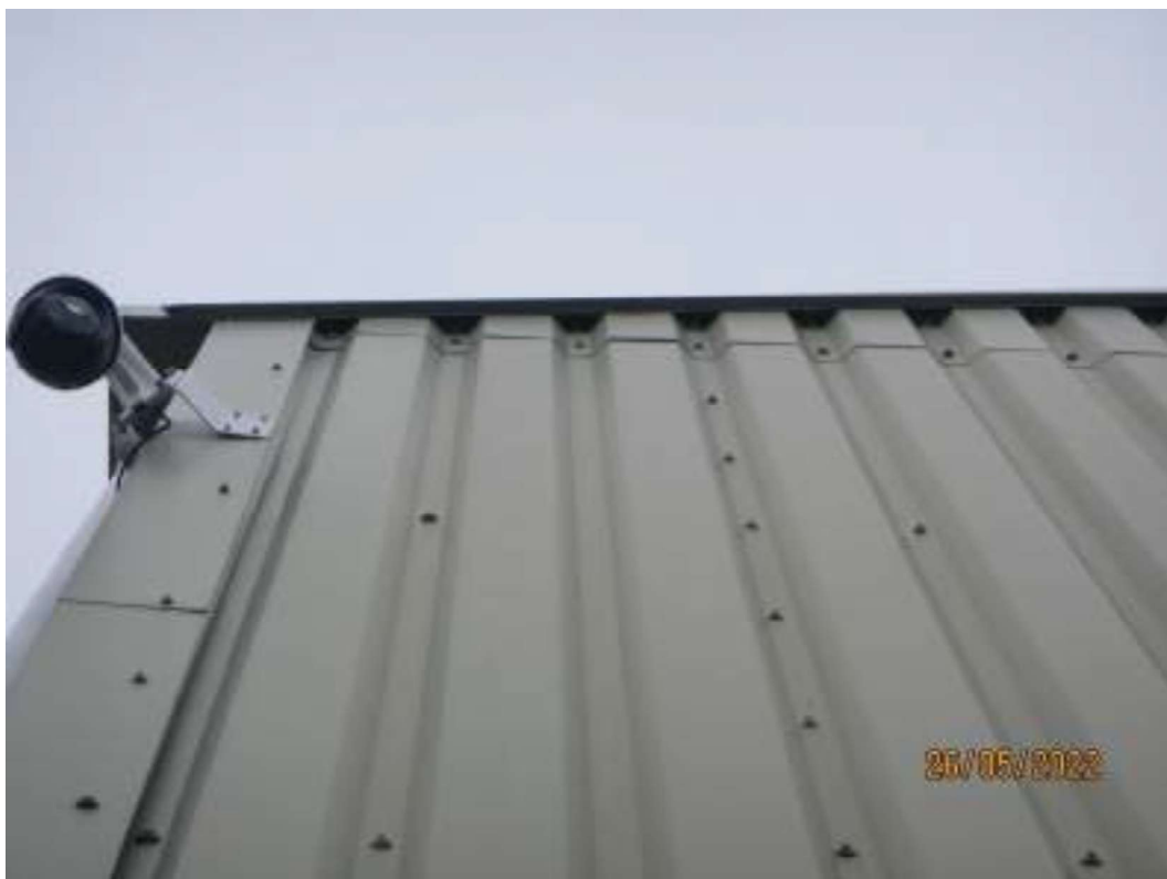
Photo 6. Example of eaves of the industrial buildings on site.
