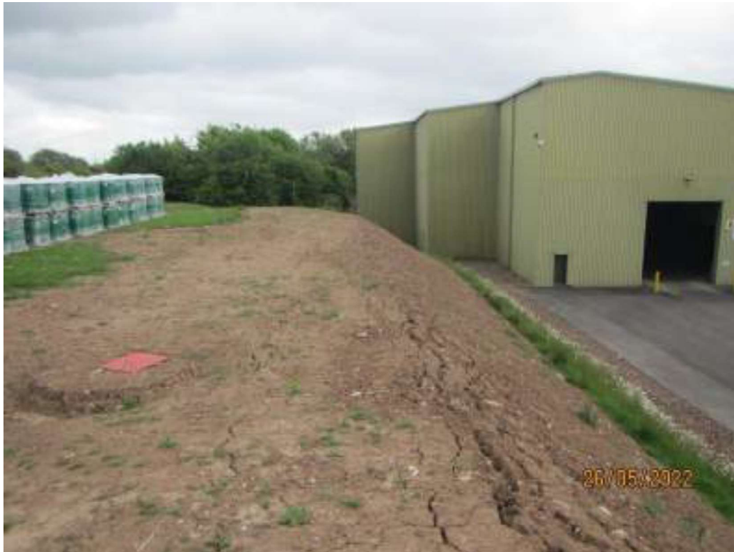
Photo 9. Looking south-east towards the building with Extension 2.
