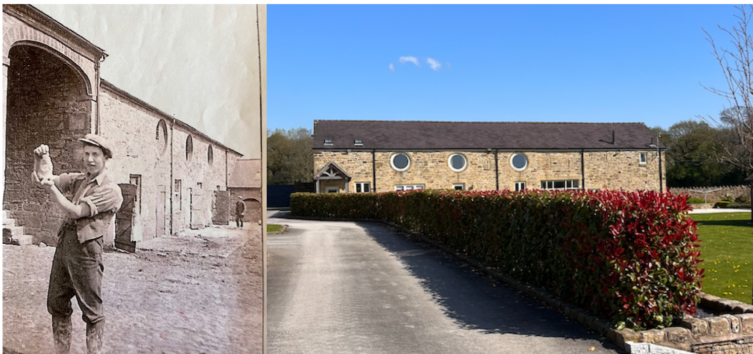
Fig 5. Left: An early photograph showing The Barn and the cart shed range, plus note the L-shape single storey return to the east. Right: the truncated converted barn today – this part is seen on the historic photograph to the left. The building is easy to identify by the stonework and the oculus windows – former hay pitching openings - at first floor level, the ground floor has been altered to accommodate the residential conversion, but single door openings are still broadly in line with the original apertures.
