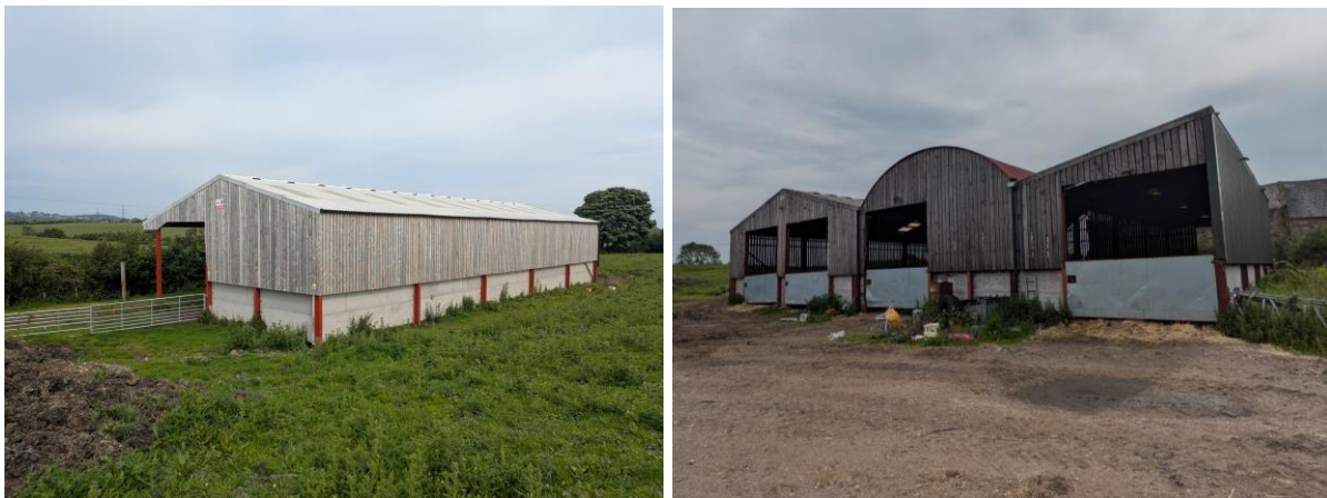
Fig. 4 & 5 – Comparative views of the new building and the existing farm barns
