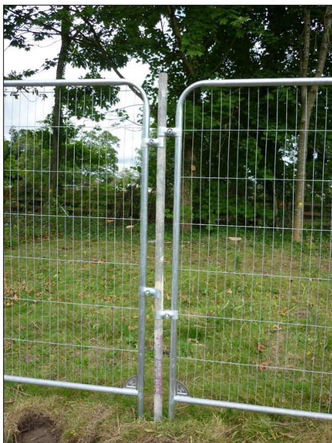
Tree Protective Fencing Specification
