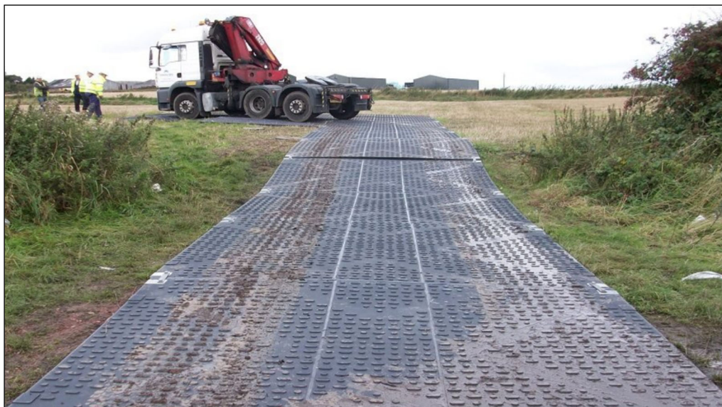
P6 – Example of ground guards used for plant access within RPA of trees
