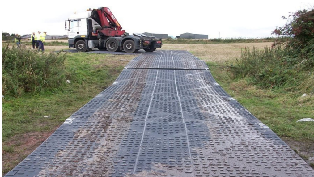
P4 – Example of ground guards used for plant access within RPA of trees
