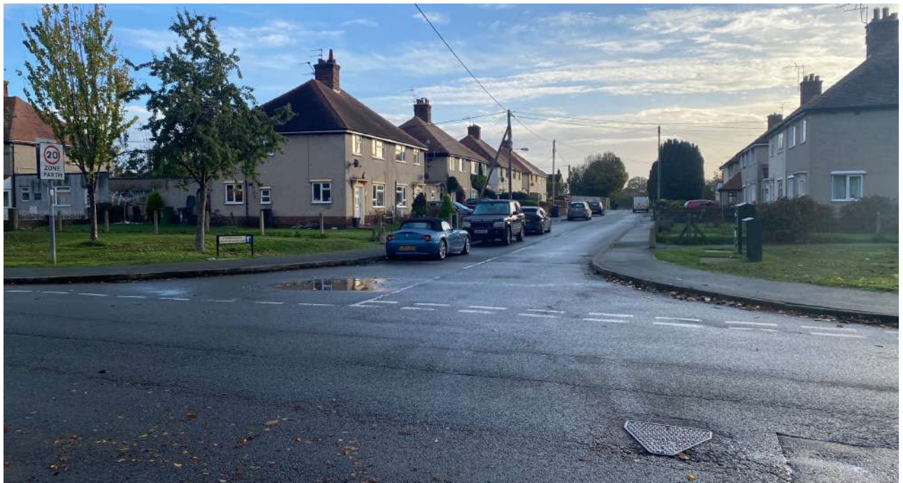
Photograph 2.6 : St Mary's Avenue – Priority Junction
