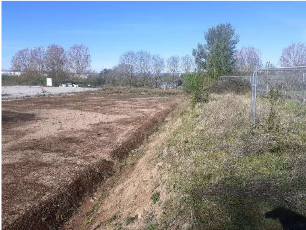
PLATE 1 SOUTH OF THE SITE – 2-3 m LOWER IN ELEVATION
