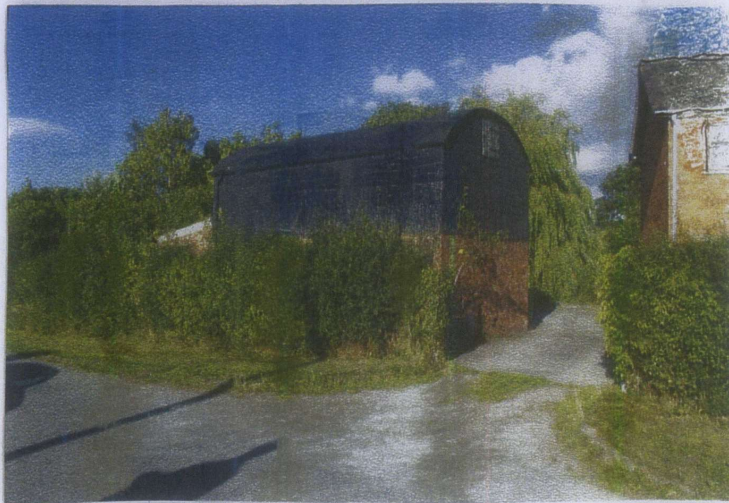
VIEW FROM CLOY LANE
