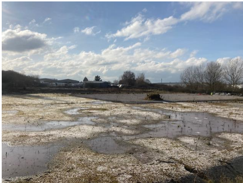
Figure 3 - view east of existing southern plot - site cleared and hardcore laid
