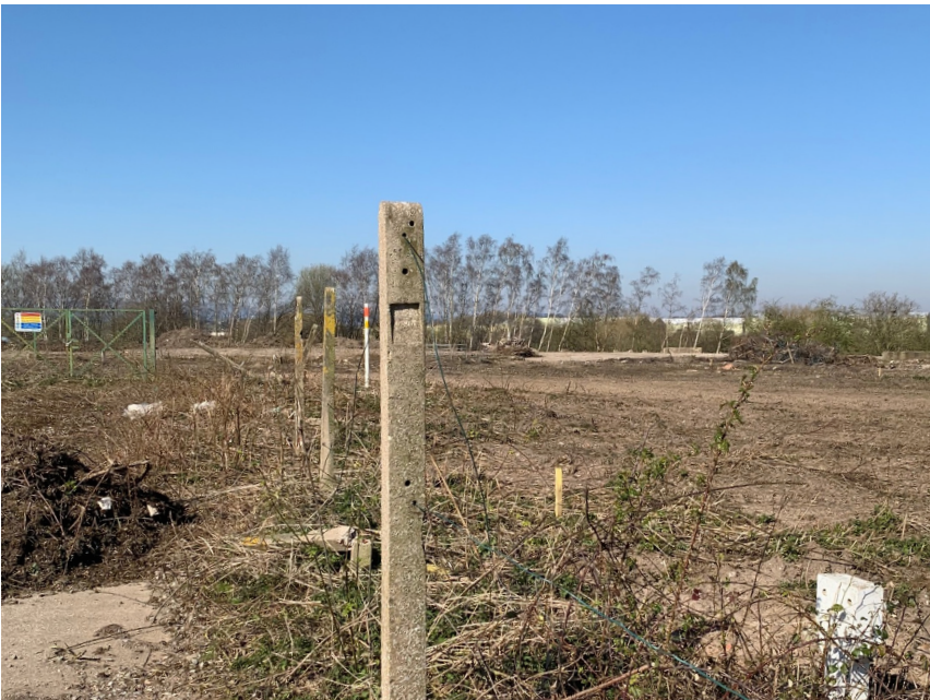
Purifier bases and hard standing - Exterior Image
