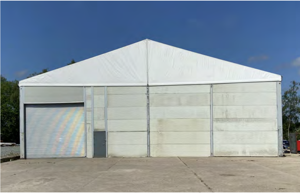
3. Building B - Front elevation as viewed from the East
