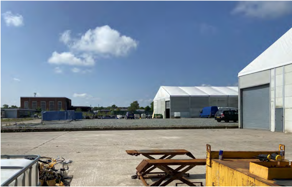
6. Building A & B - As viewed from the North with Training Centre of WWU in background
