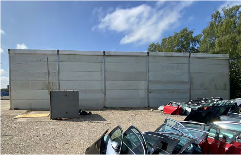
4. Building B - Side elevation as viewed from the North
