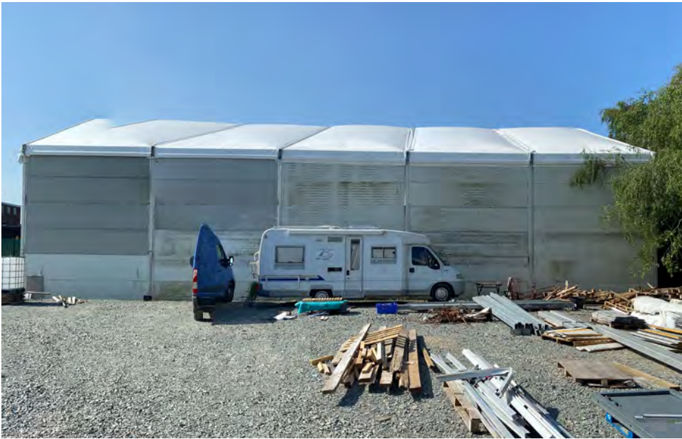
2. Building A - Side elevation as viewed from the North
