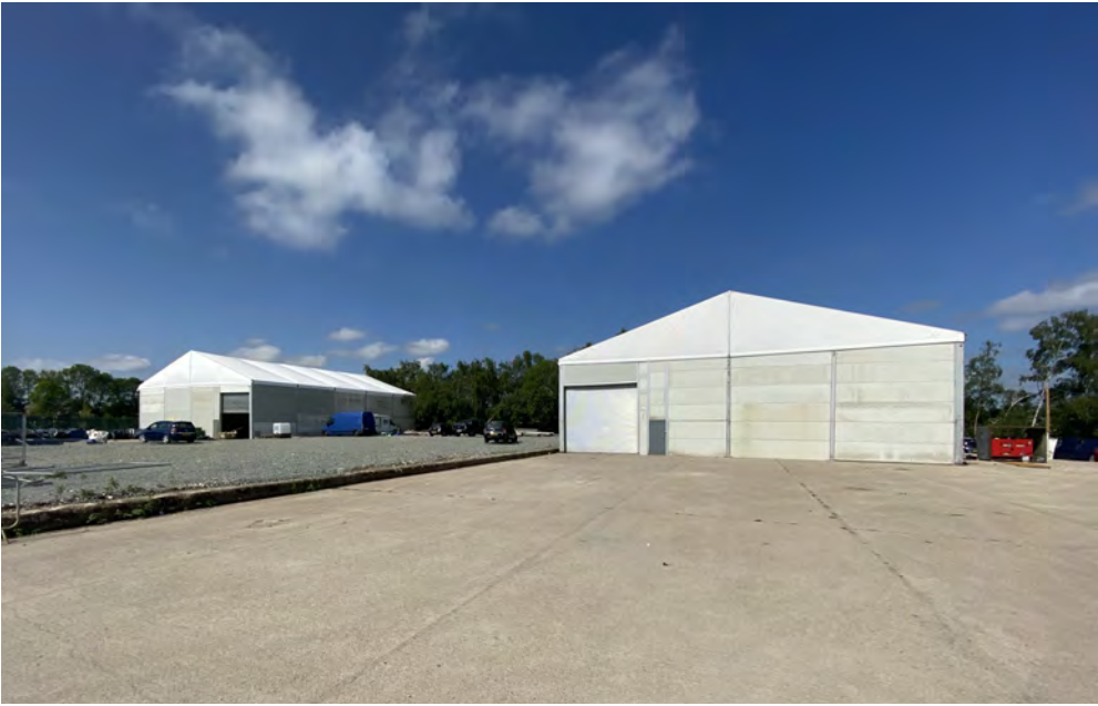
5. Building A & B - As viewed from the East
