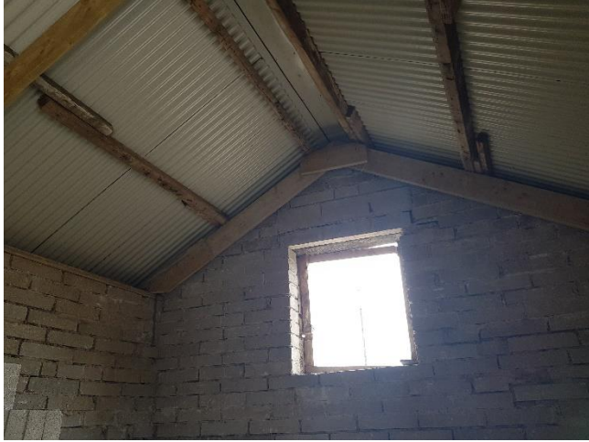
Interior of barn.
