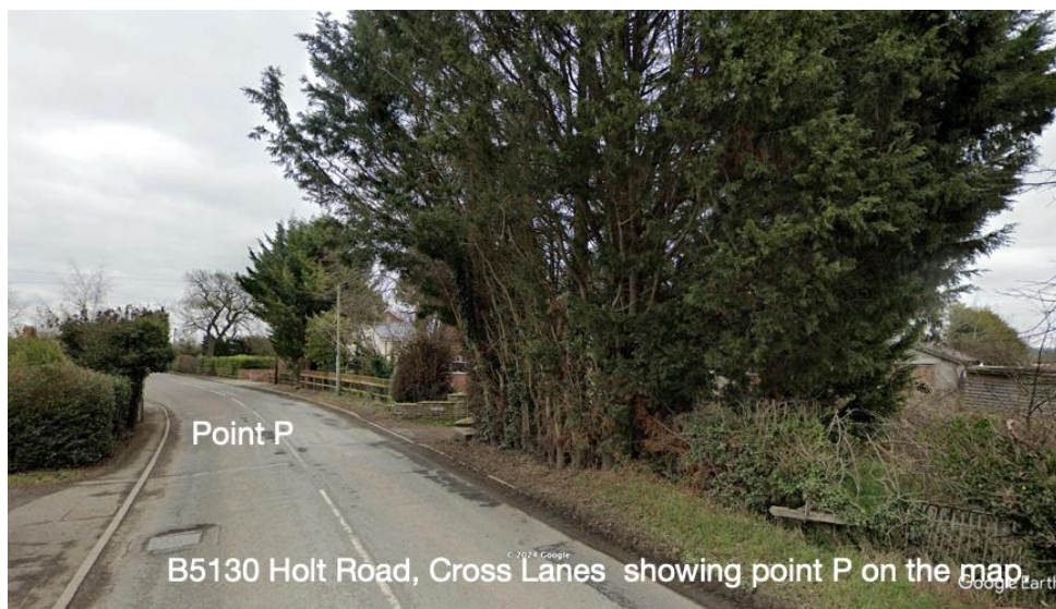
Photograph 2. View along Holt Road looking towards Point P on Map 1 at the vulnerable point showing the narrow footpath.
