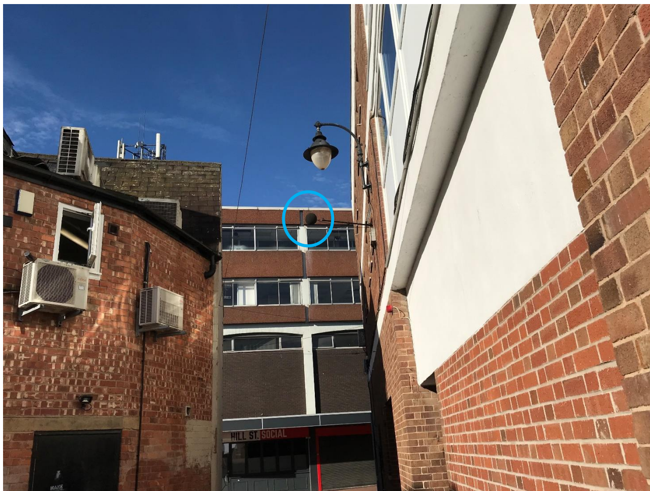
Figure 3: Photograph Showing Monitoring Position 3
