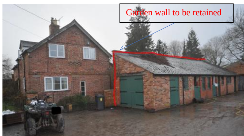
The Gardener's Cottage, with adjacent stables to be demolished but retaining garden wall
