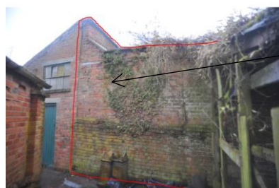
west flank wall
