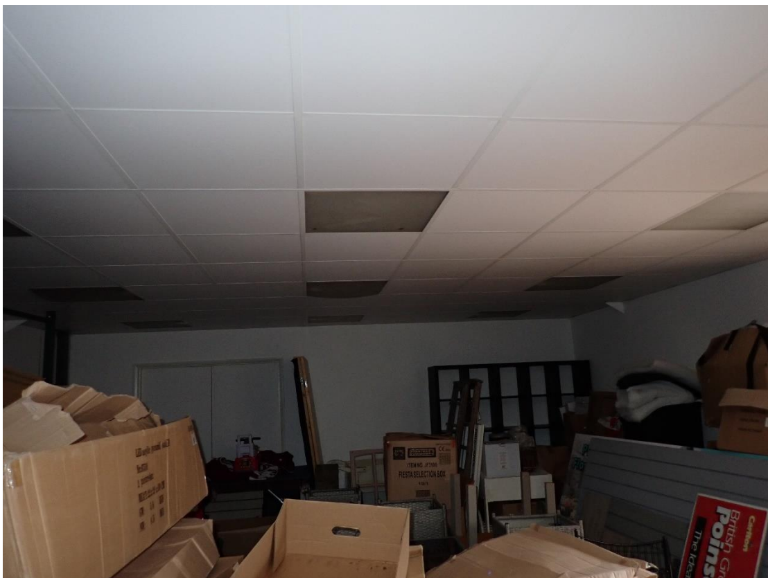
Photograph 4 – south to north across internal space within building 1, false ceiling and no roof void.
