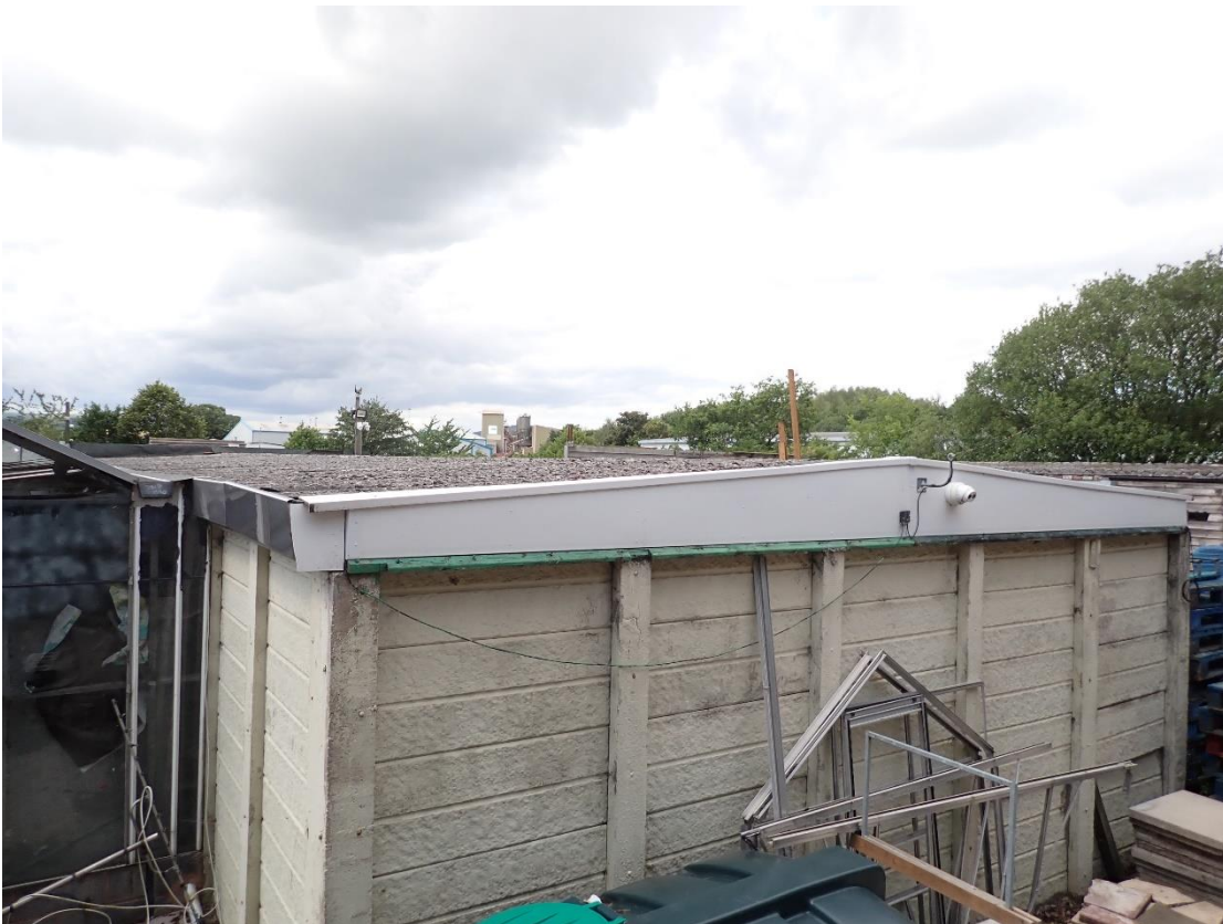
Photograph 6 – northeast aspect of building 2 with asbestos flat roof.
