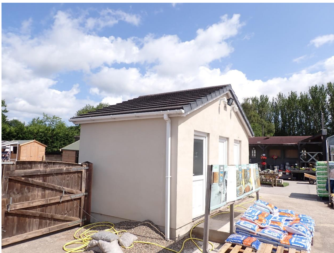
Photograph 11 – negligible WC structure on site due to be retained as part of proposed plans.
