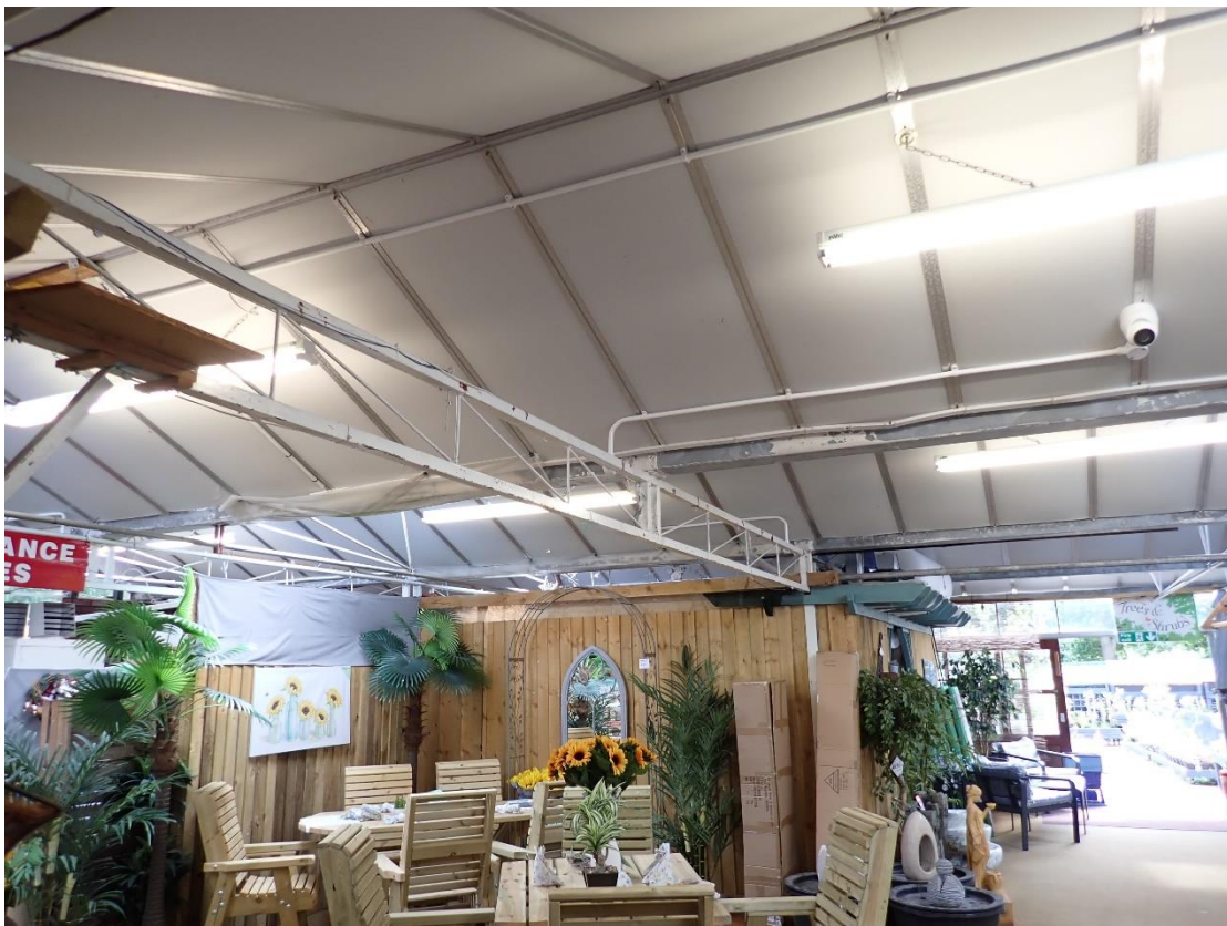
Photograph 10 – north to south across garden centre showing single lined pitched roof.
