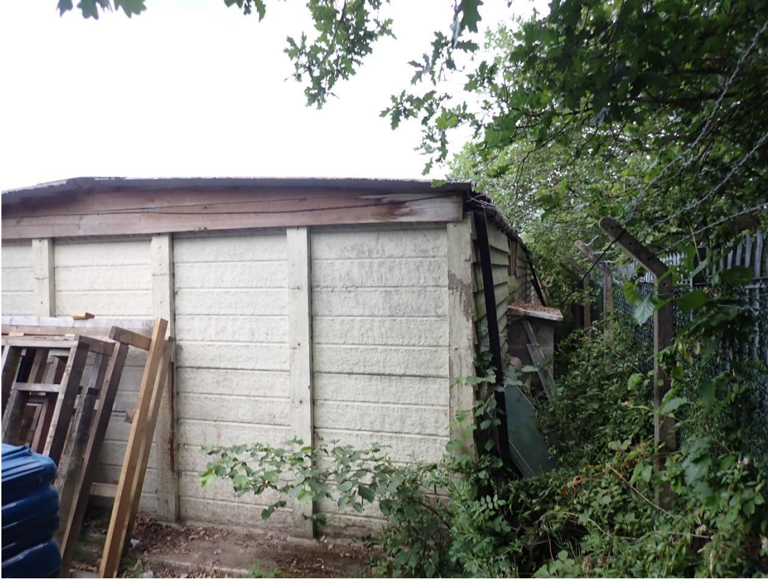
Photograph 1 – northeast aspect of building 1 on site.
