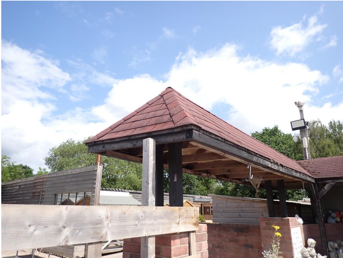
Photograph 7 – roof structure extending from west aspect of building 2.
