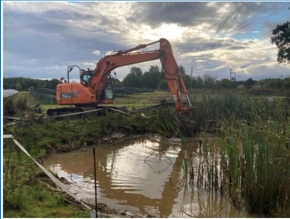
Desilting in progress (06/10/21)
