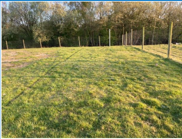
Example of stock proof fencing installed around Pond 3 (19/04/21)
