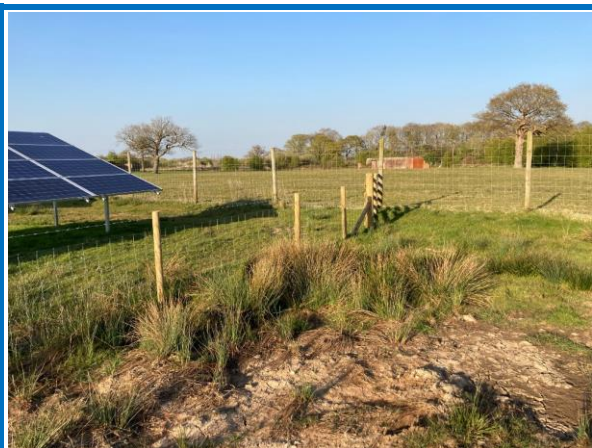
Example of stock proof fencing installed around Pond 1 (19/04/21)
