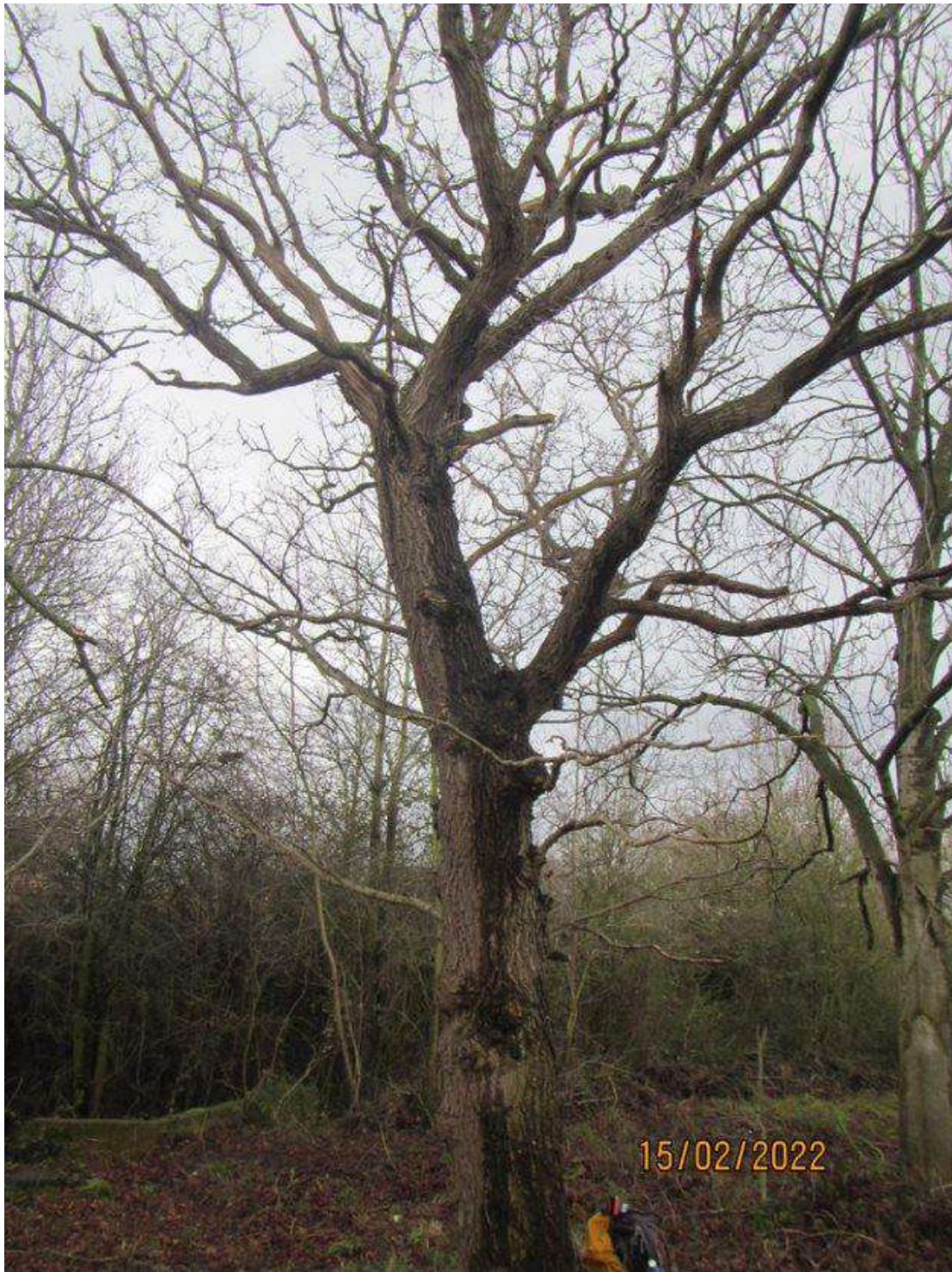
Photograph 4 – T3 showing tear-out at base of crown.
