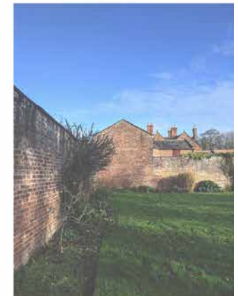
Gable end of west wing from garden
