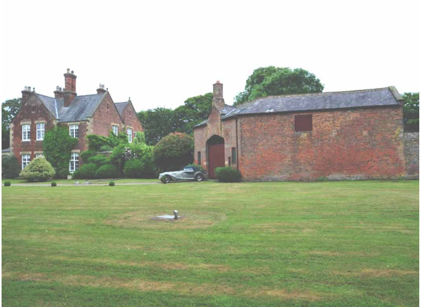
Cedar Hall (Left) and Stable block (Right) Source: Richard K Morriss & Associates
