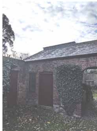
Rear of stable from Cedar Hall
