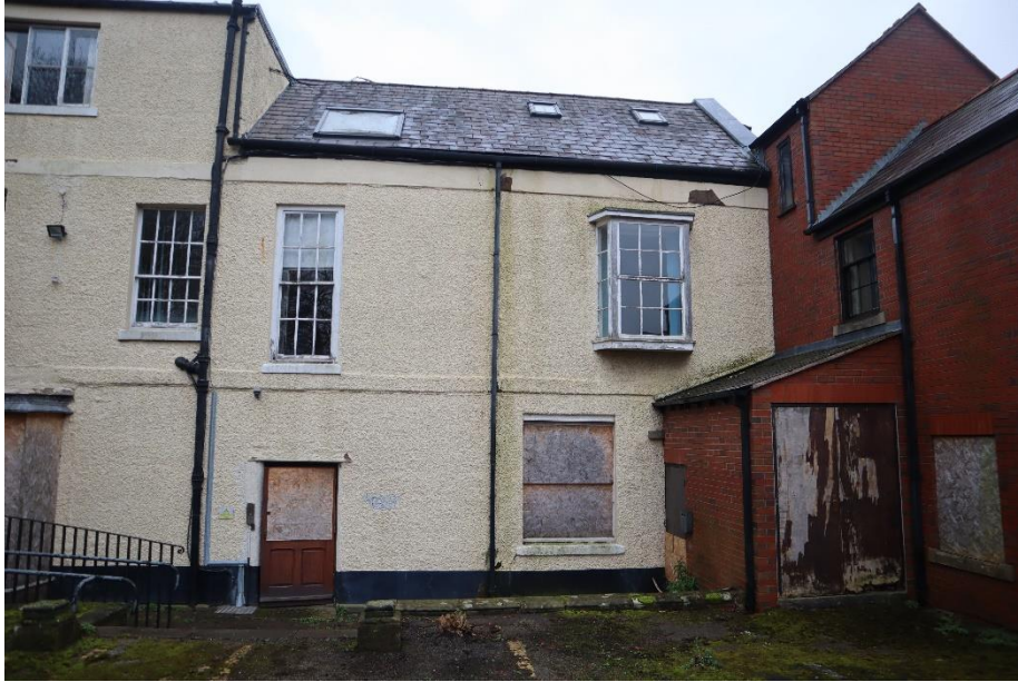
Figure 18 – Rear of 23 Chester Street
