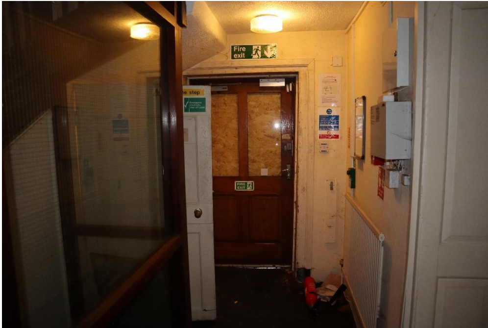
Figure 47 – Ground floor stairwell of 23 Chester Street
