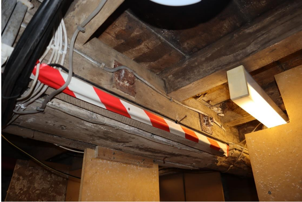
Figure 61 – Basement of 23 Chester Street
