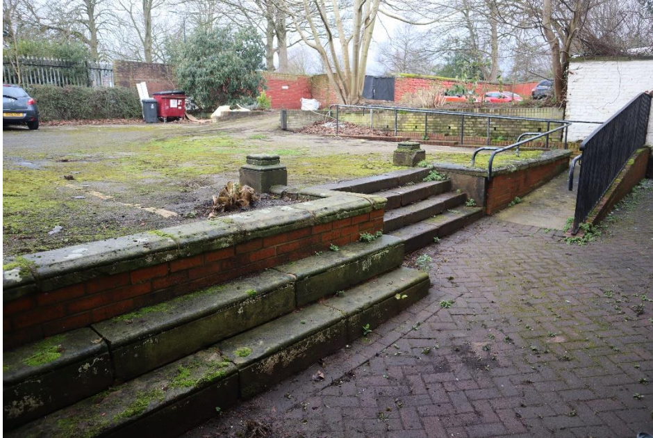
Figure 20 – Rear of 23 Chester Street
