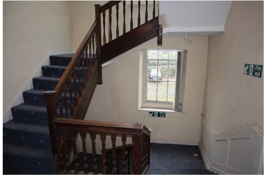
Figure 93 – First floor stairwell of 23 Chester Street
