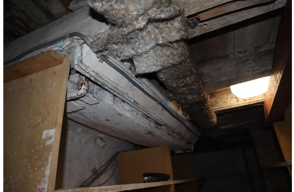
Figure 56 – Basement of 23 Chester Street
