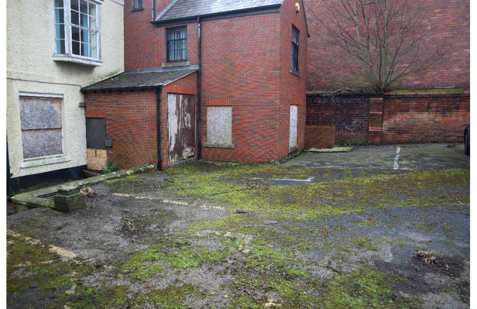
Figure 21 – Rear of 23 Chester Street
