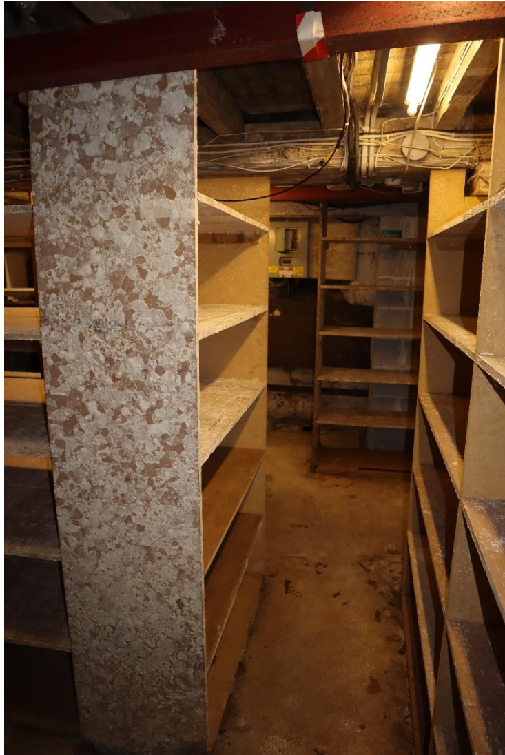
Figure 55 – Basement of 23 Chester Street
