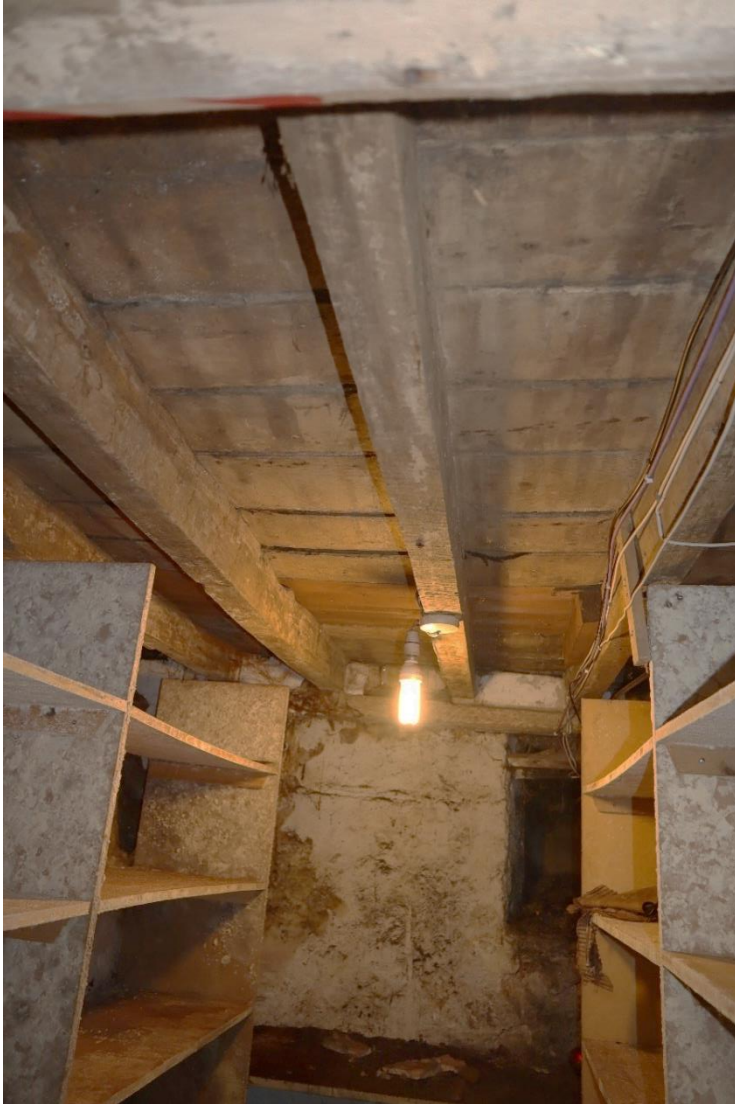
Figure 53 – Basement of 23 Chester Street
