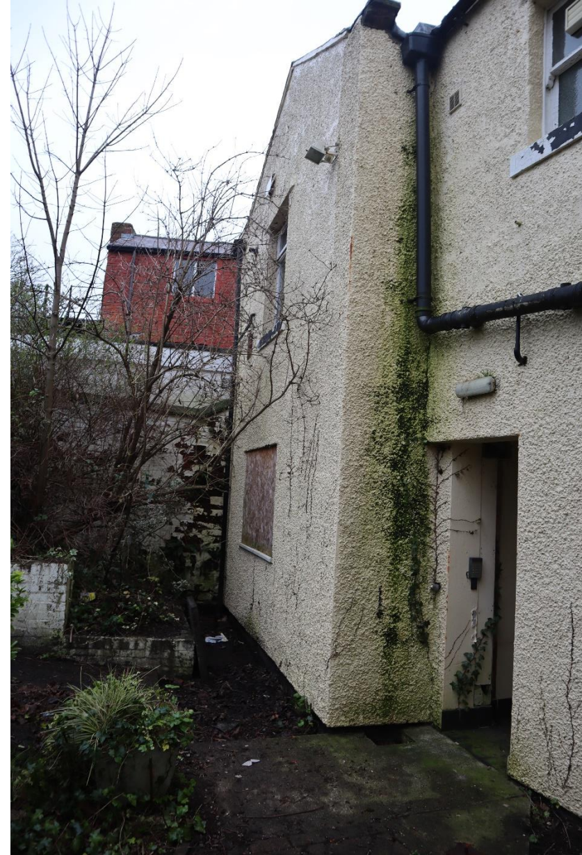
Figure 27 – Rear of 24 Chester Street
