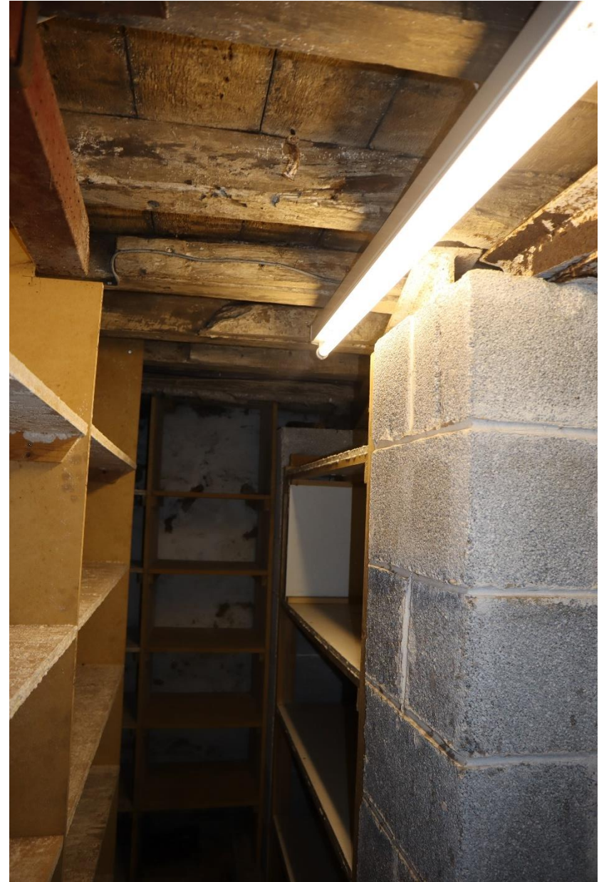
Figure 62 – Basement of 23 Chester Street
