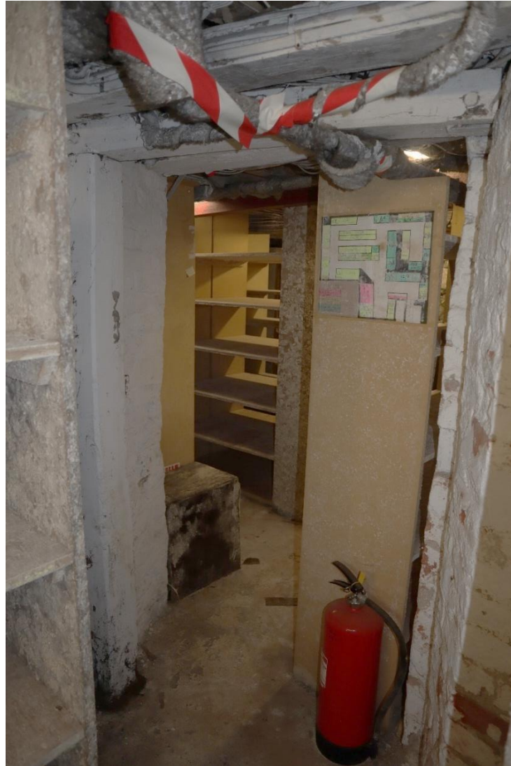
Figure 54 – Basement of 23 Chester Street
