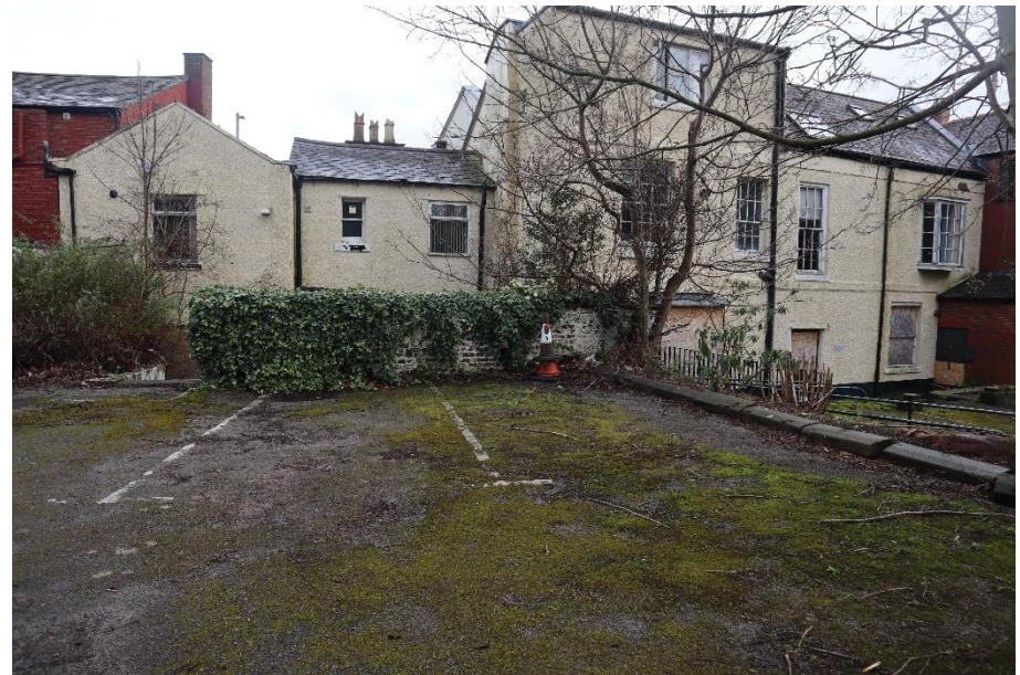
Figure 29 – Rear of 24 Chester Street
