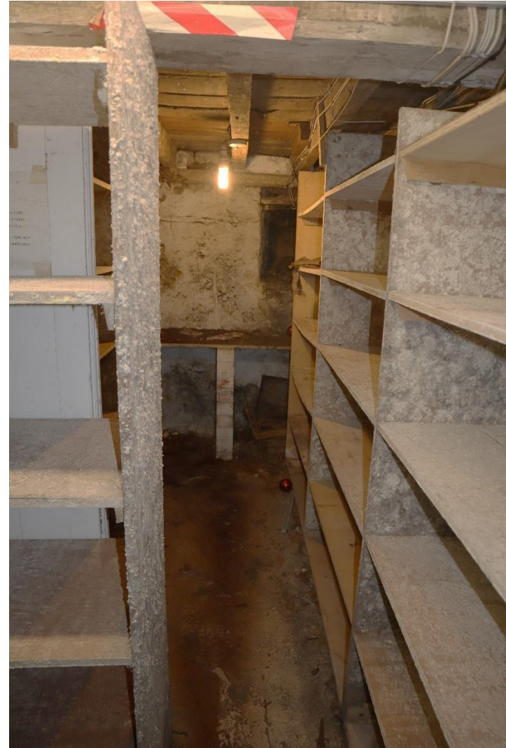
Figure 52 – Basement of 23 Chester Street
