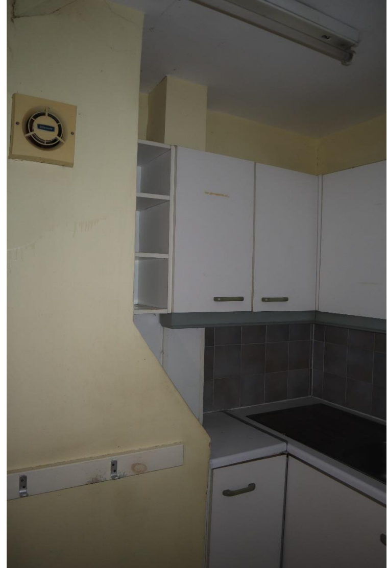
Figure 162 – Rear second floor rooms of 23 Chester Street
