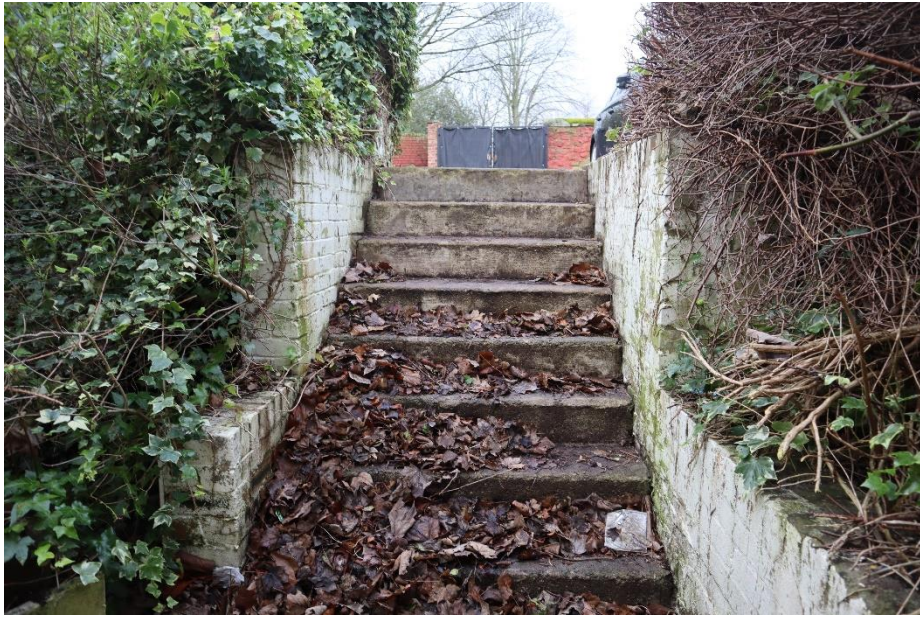
Figure 28 – Rear of 24 Chester Street
