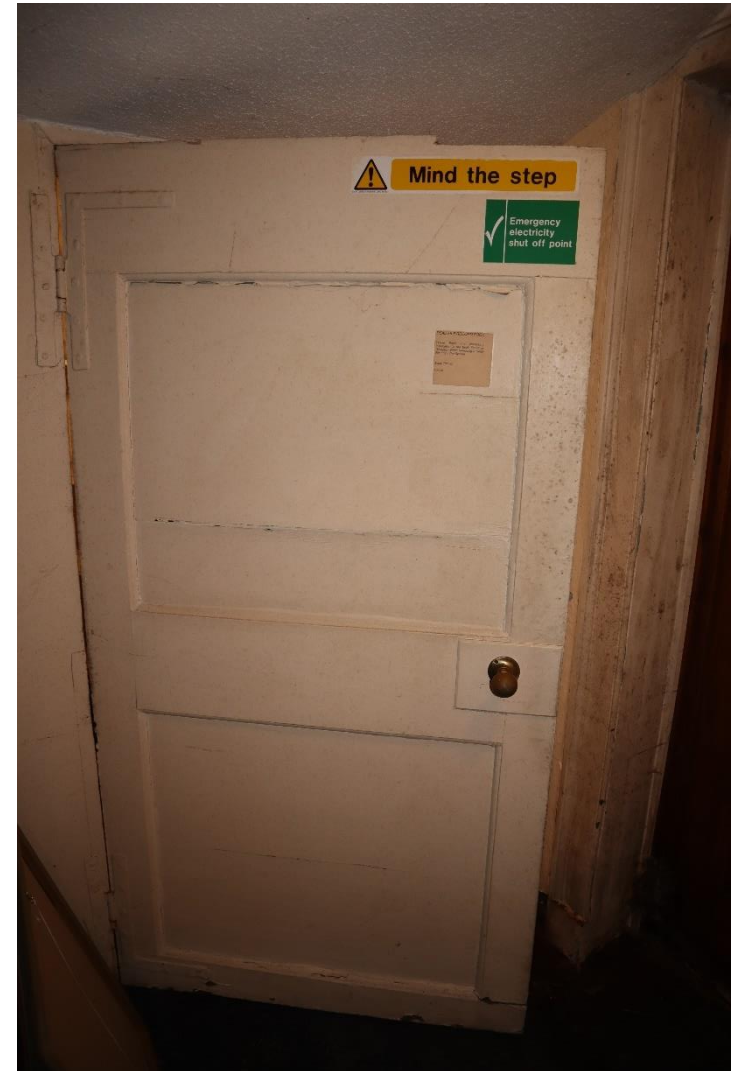
Figure 48 – Basement of 23 Chester Street
