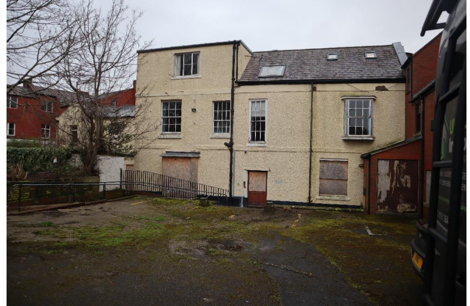
Figure 19 – Rear of 23 Chester Street
