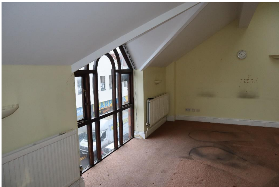
Figure 155 – Room 15 of 23 Chester Street
