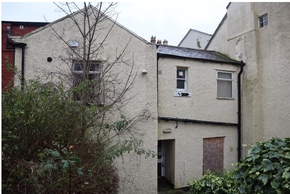
Figure 22 – Rear of 24 Chester Street
