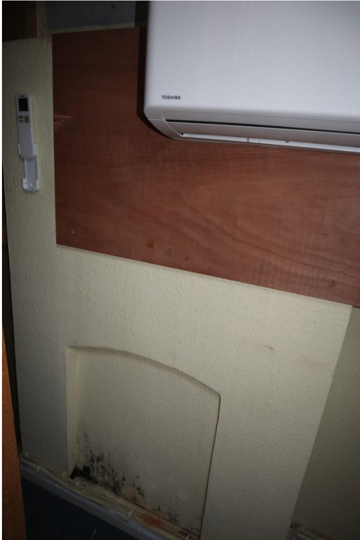
Figure 167 – Rear second floor rooms of 23 Chester Street
