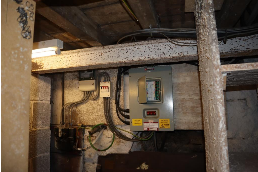
Figure 59 – Basement of 23 Chester Street
