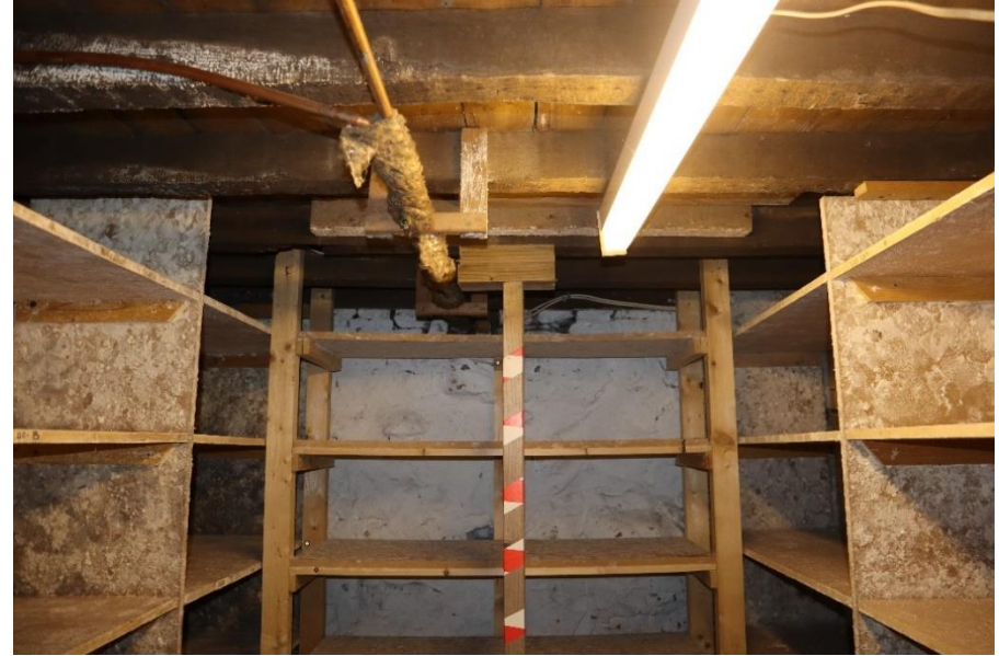
Figure 60 – Basement of 23 Chester Street
