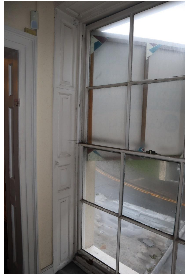
Figure 99 – First floor stairwell of 23 Chester Street
