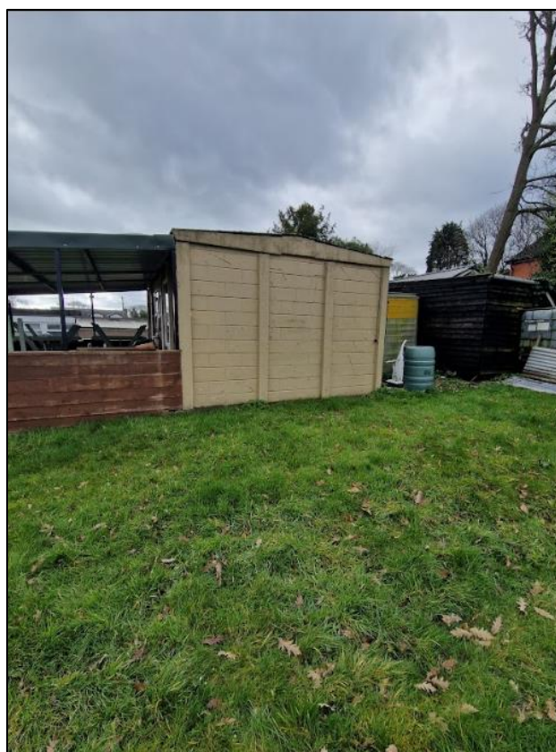
Plate 4 – Building 2 viewed from the north
