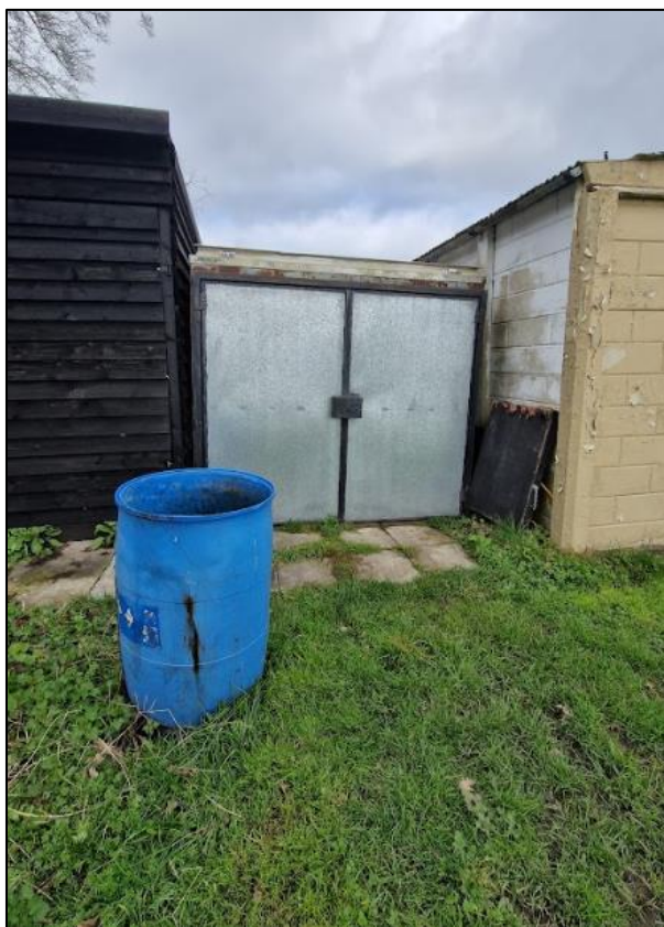
Plate 5 – Building 3 Storage container.
