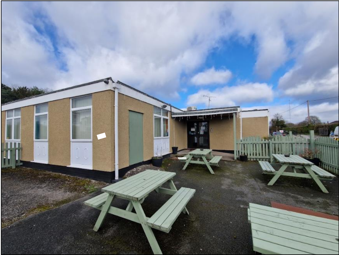
Plate 1 – Building B1 viewed from the southwest
