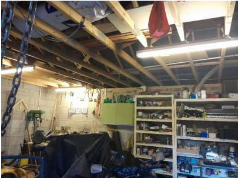
Figure 10 - overview of the interior of B1.
