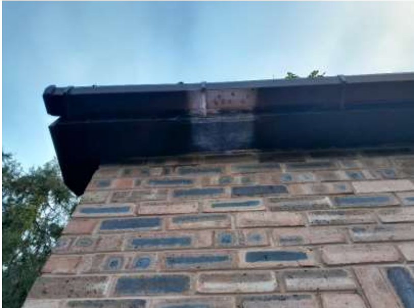
Figure 9 - the soffits in good condition.
