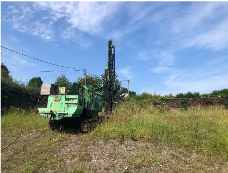
Rig on Bh 3
