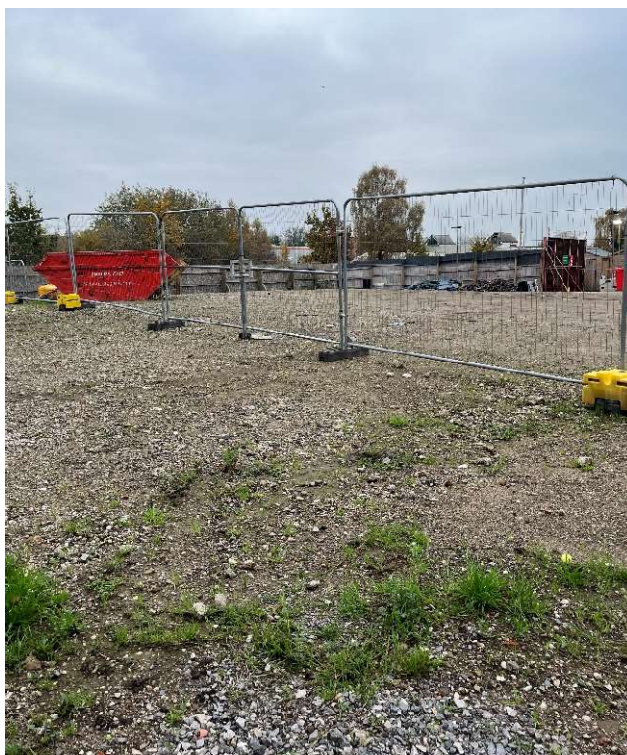
Figure 3 – View of existing site condition
