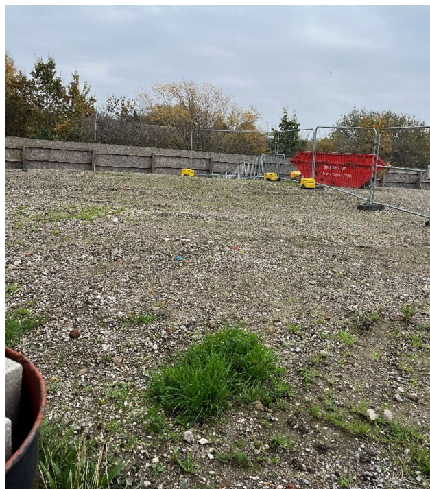
Figure 2 – View of existing site condition
