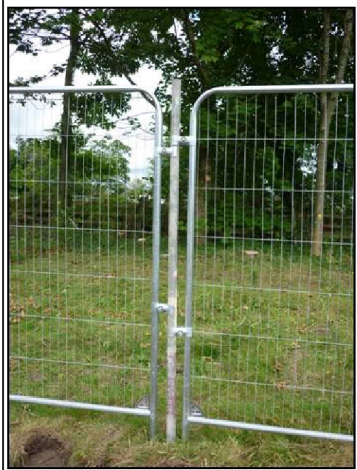
Tree Protective Fencing Specification
