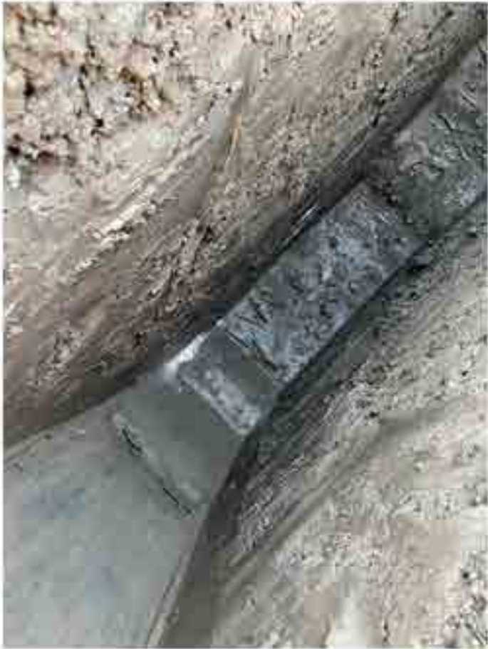
Concrete utility at base
