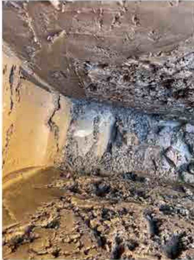
Concrete utility at base 1
