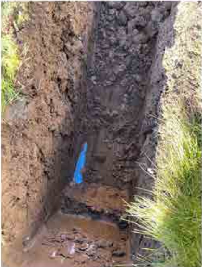
TP103 utility and pit
