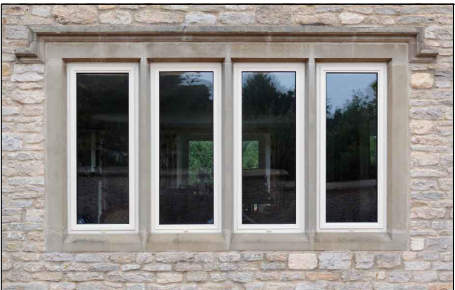
Reinstated stone mullions with Aluminum windows (Off White).
