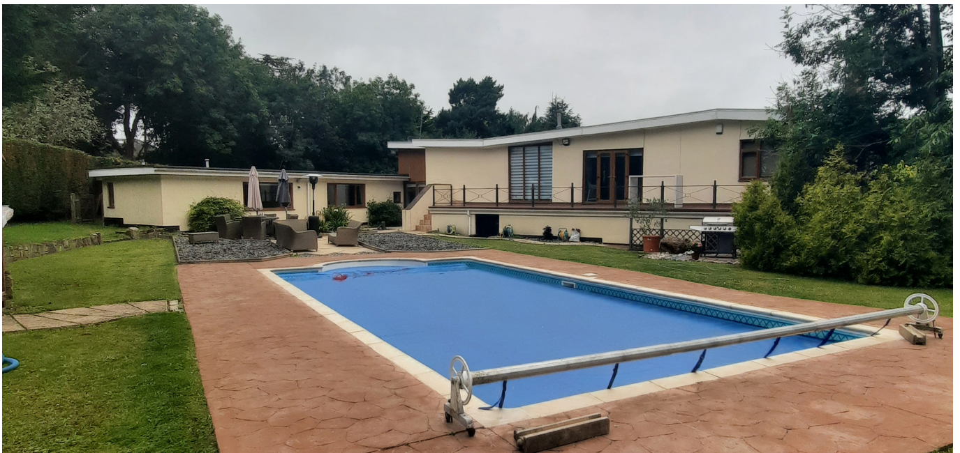
Image showing the current rear elevation of Pine Ridge
