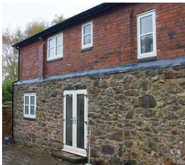
Figure 2 Rear elevation of the property, showing the random rubble stone wall which is to be opened up and where possible the stone reclaimed and reused within the extension. Grey brick soldier courses at the heads and cills of door and window openings will be continued within the extension.
