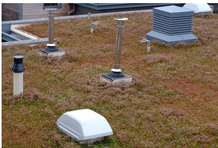
Figure 1 BauderGreen XF 301 lightweight sedum system on The Walnuts School, Hazeley
