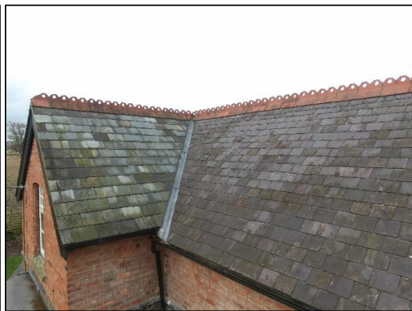
Figure 10: The tight-fitting slates and ridge tiles.
