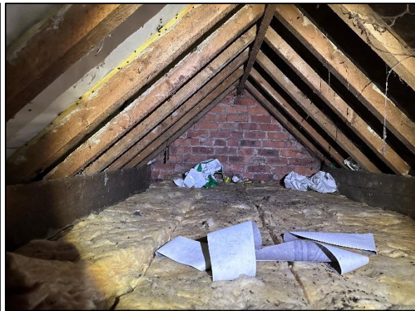
Figure 4: The roof void within the building.
