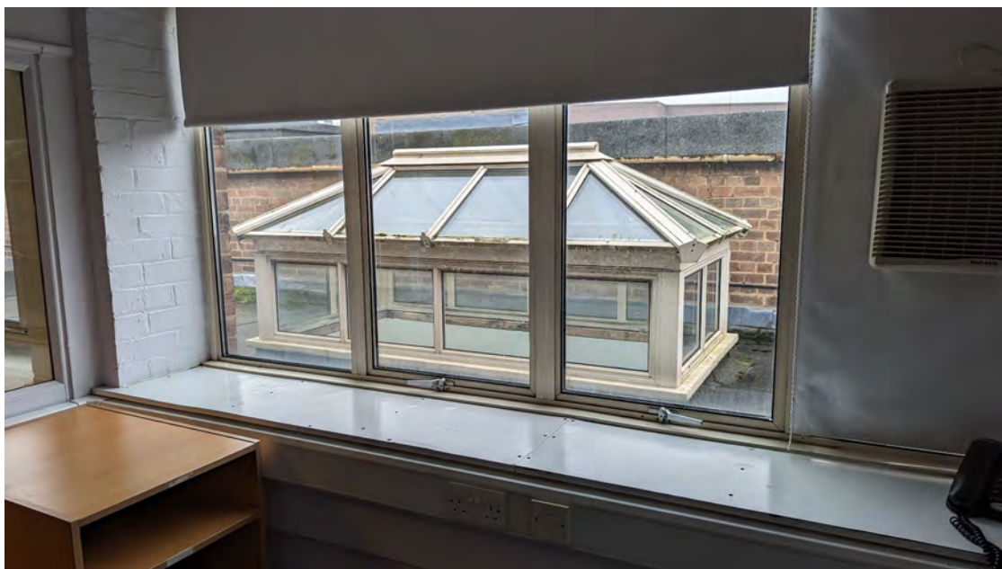
Plate 4: Lantern light over corridor
