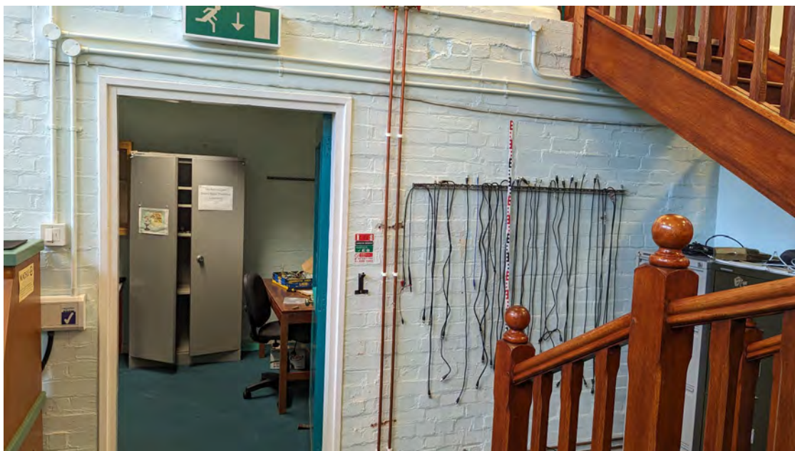
Plate 17: Room C36a, doorway to C36
