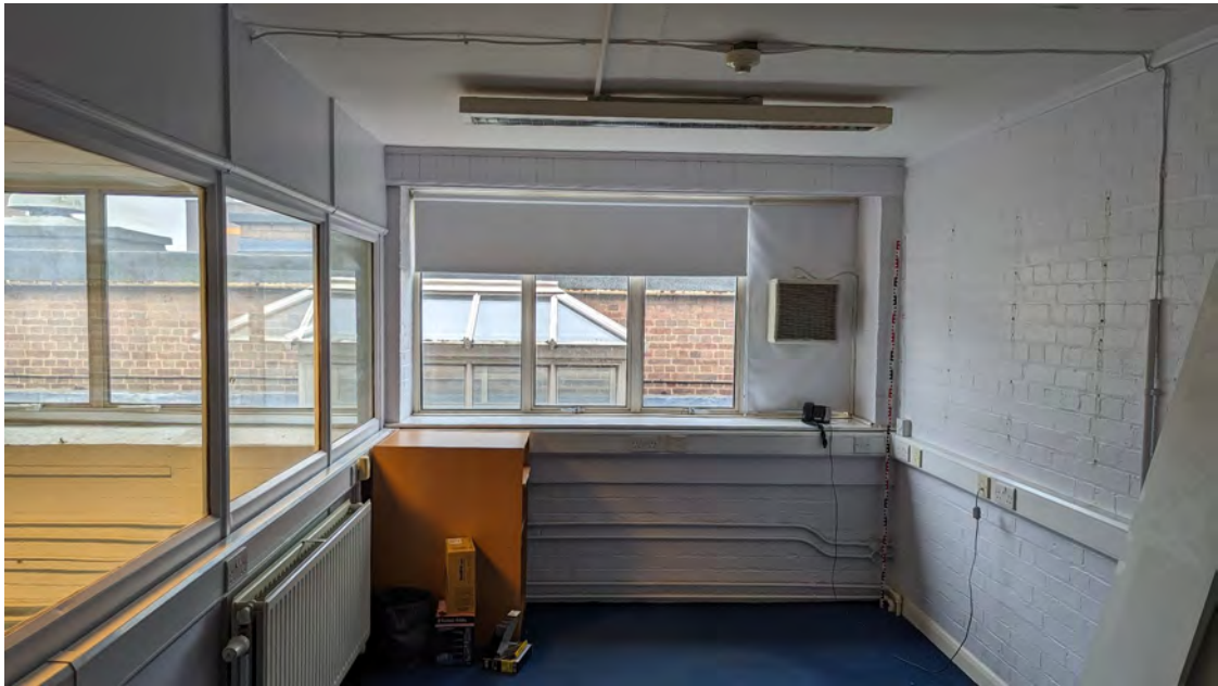
Plate 24: Room C36 first floor, looking southwest
