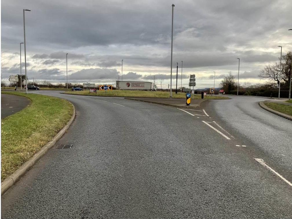
6.1 General view looking east on Abenbury Way towards Bryn Lane Roundabout.
