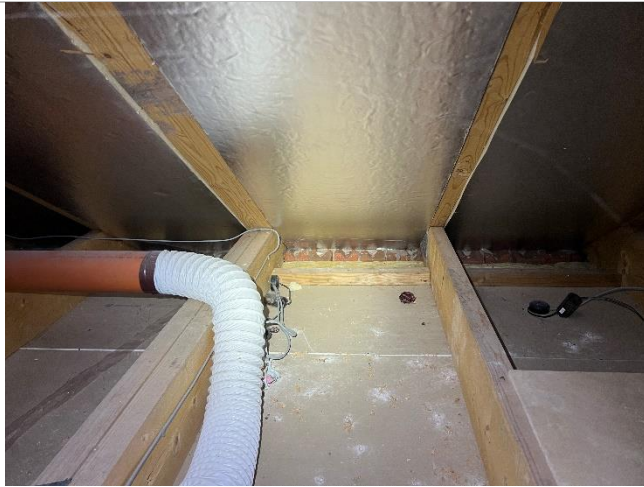
Interior eaves space.
