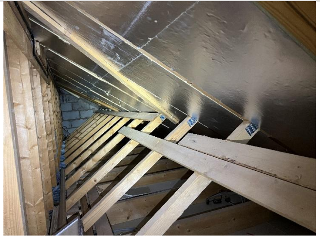
Interior eaves space.
