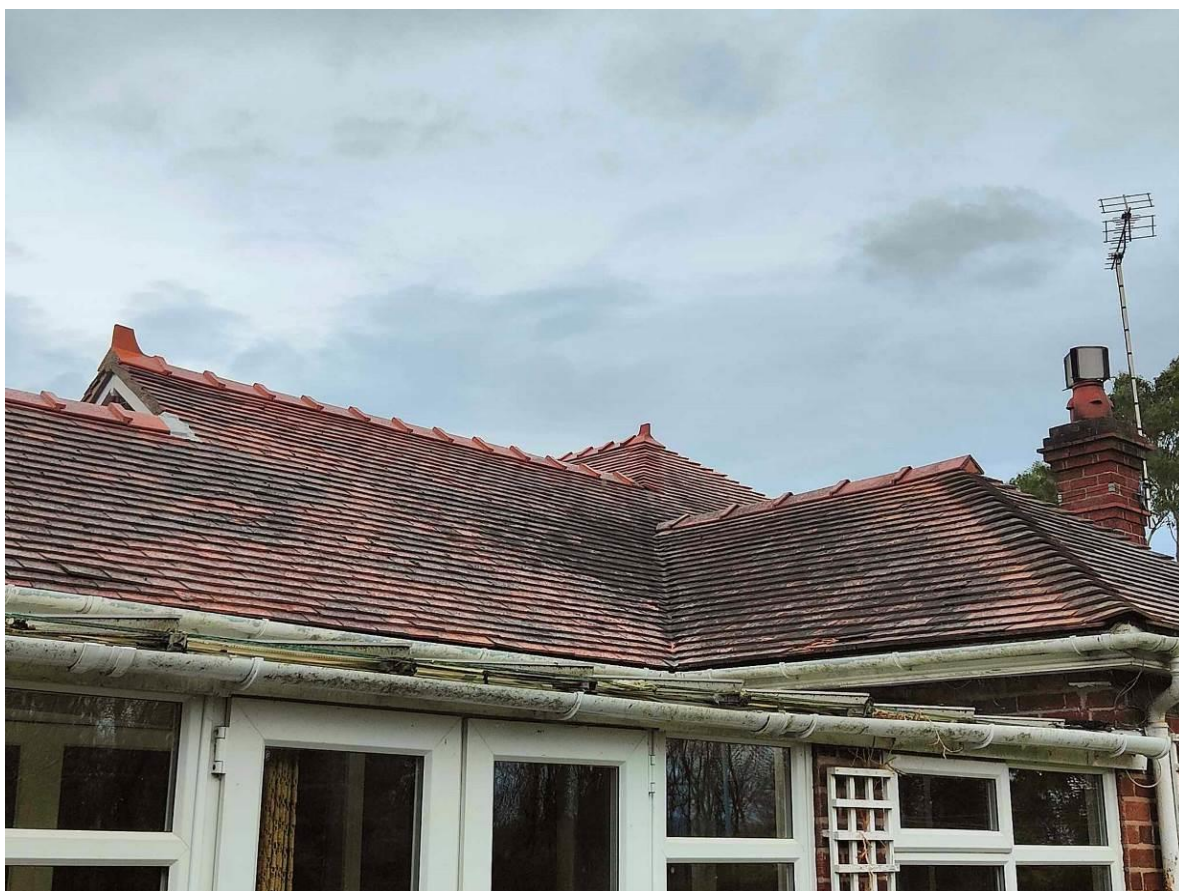
Roof of building in good condition.
