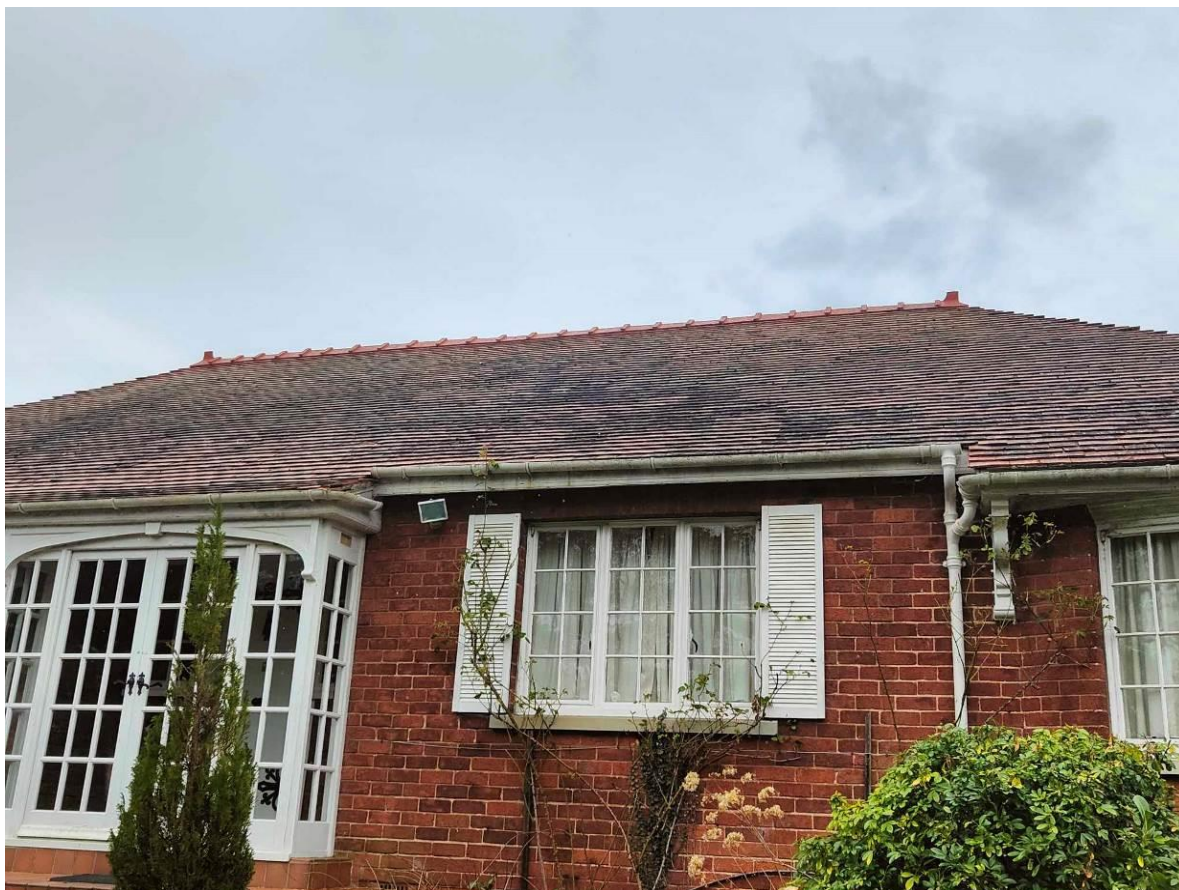
Roof of property.
