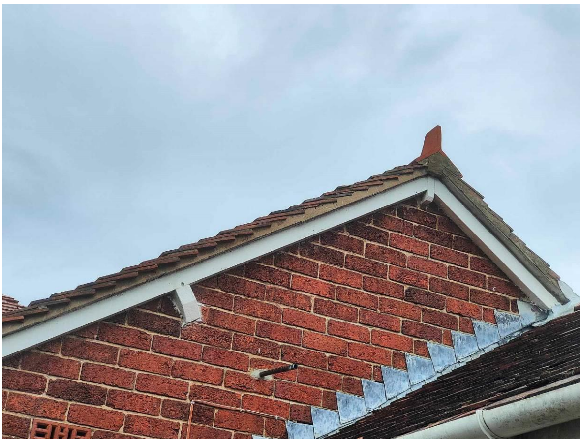
Sealed slate edges.
