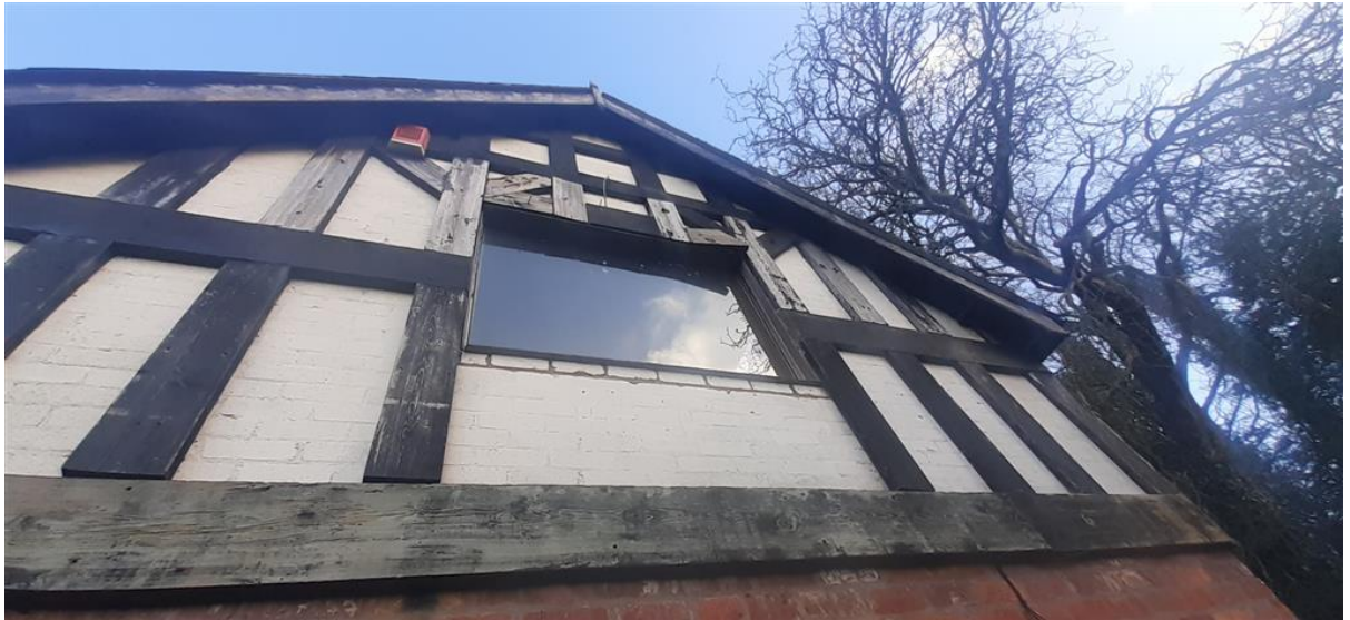
Plate 7: View of the eastern elevation – note the eaves all around the building appear tight and lack ingress points.
