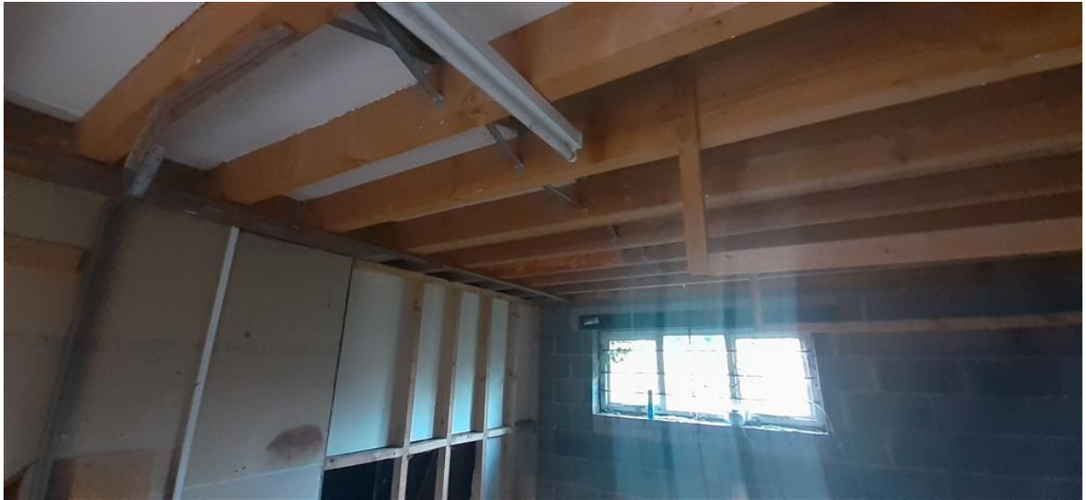
Plate 4: View of the ground floor garage.
