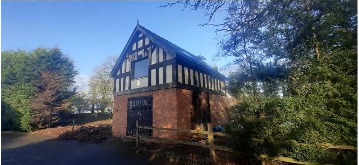
Plate 1: View of the coach house – north-eastern elevation.
