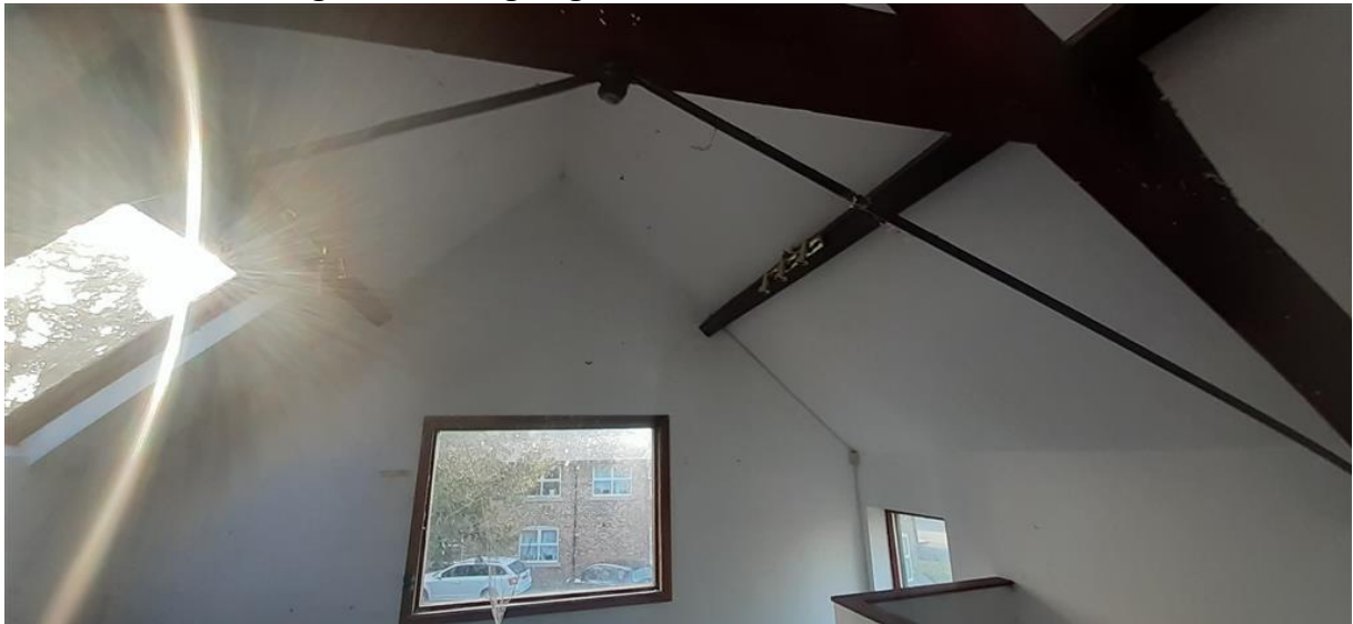
Plate 5: View of first floor – note the lack of a roof void and the well-illuminated environment from natural daylight.
