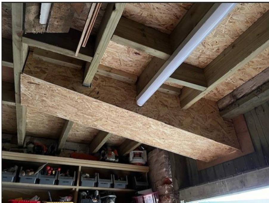
Figure 12. Sloped tunnel into loft space from letterbox access
