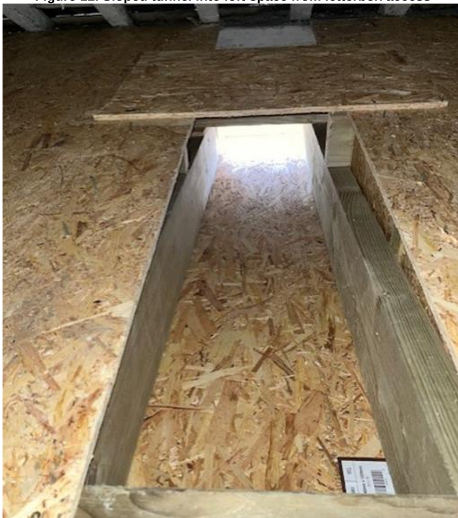
Figure 13. Clear tunnel entrance into loft
