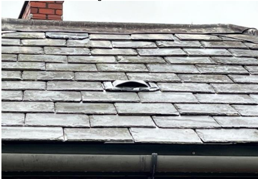
Figure 15. Crevice bat access built into roof
