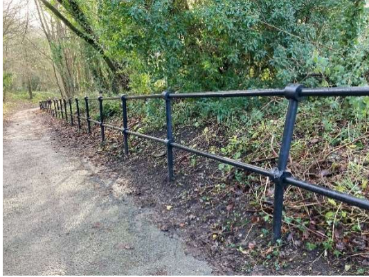
Figure 1: Example of the existing railing
