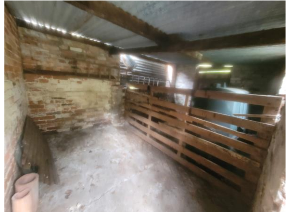
P12: Lean-to interior: looking N
