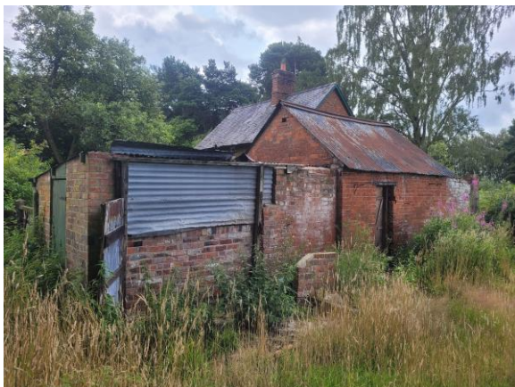
P9: NE (end) + NW (side) elevations: looking SW
