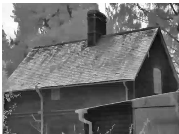
P17: 3 rd thermal imaging camera view (NW gable)
