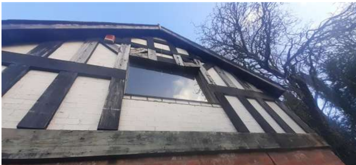
Plate 7: View of the eastern elevation – note the eaves all around the building appear tight and lack ingress points.
