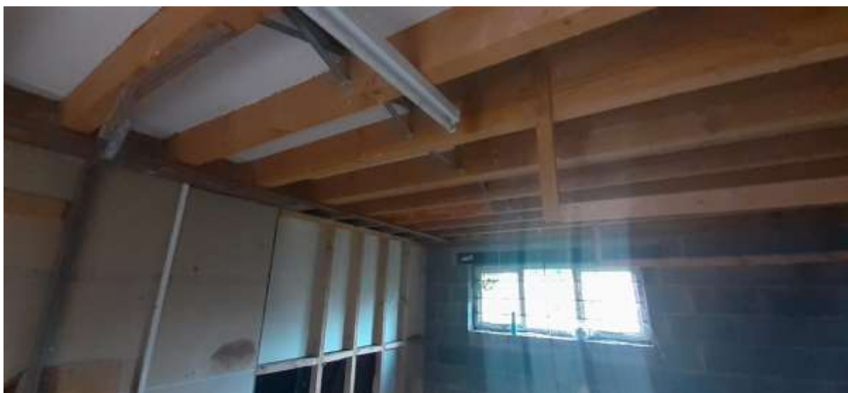
Plate 4: View of the ground floor garage.
