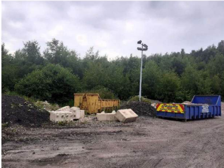
Figure 18 Hardstanding & Skips (North East of the Site)
