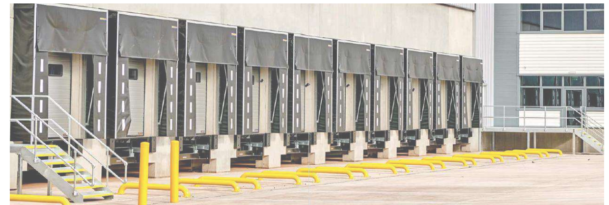
Provision of dock levelling equipment is key to the determination of site levels and floor levels
