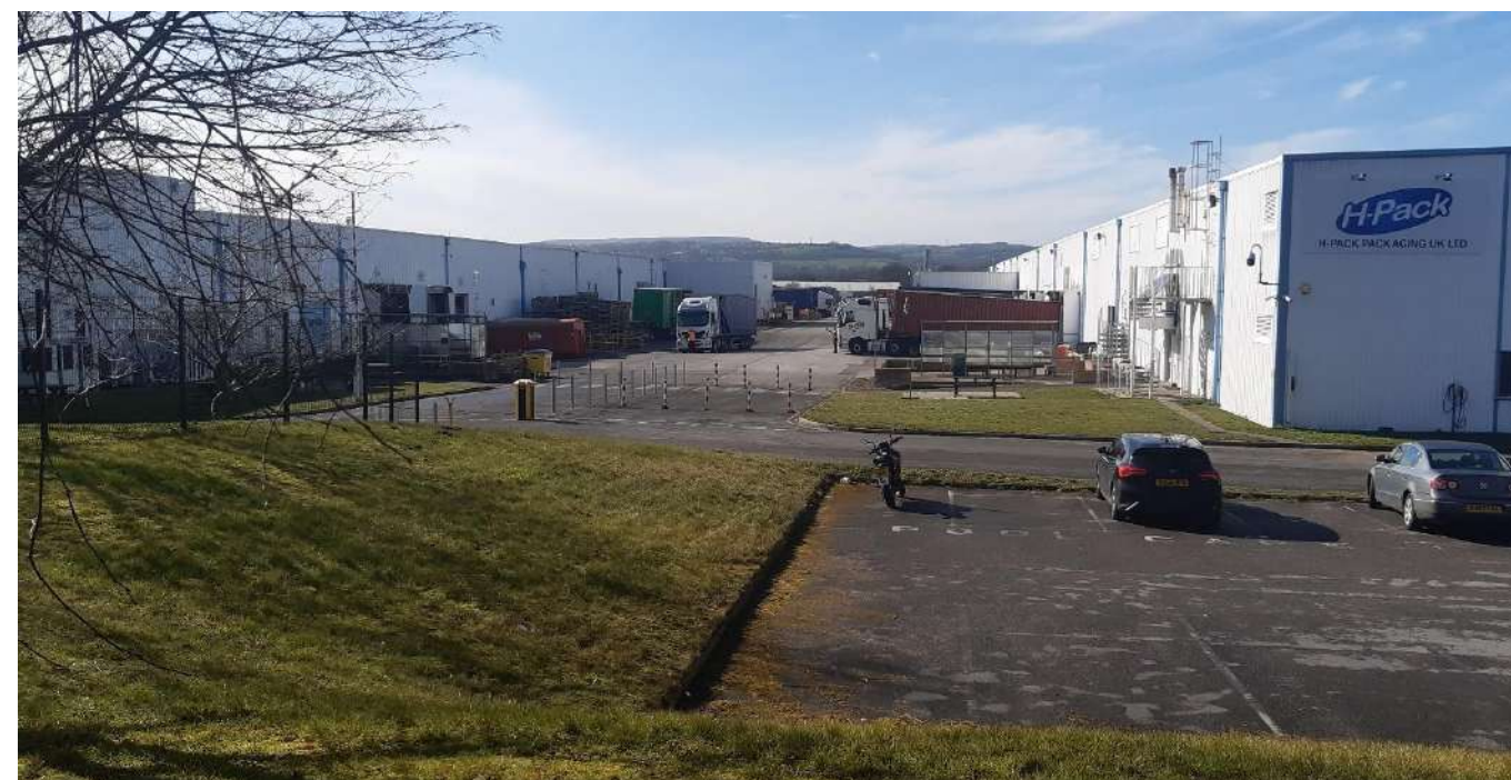
View southwest towards the shared service area.
