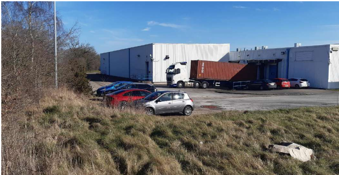
Existing facility, viewed from the northern boundary.
