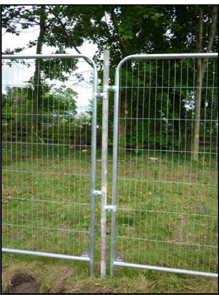
Tree Protective Fencing Specification
