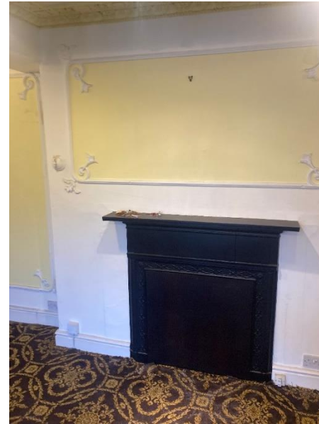
FIGURE 7 - DETAIL TO THE FIRST FLOOR OF 23 CHESTER STREET © LIATH HERITAGE 2024
