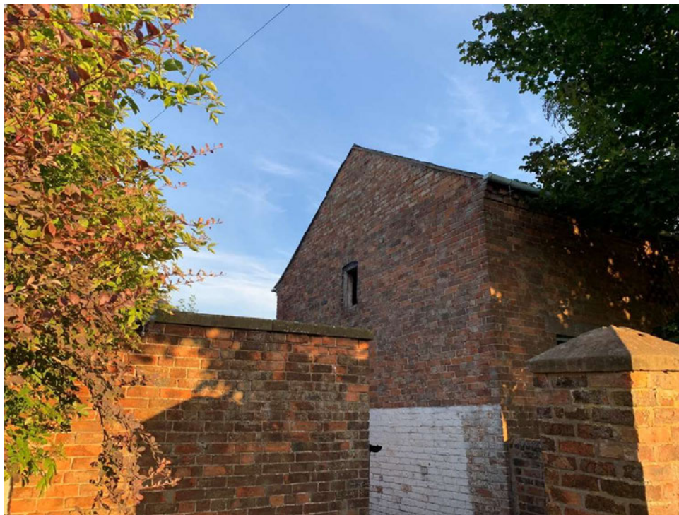
Photograph 8: Building C (eastern gable end)
