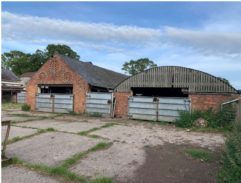
Photograph 10: Building E (left) & F (right)
