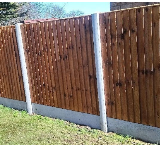
Example of fencing
