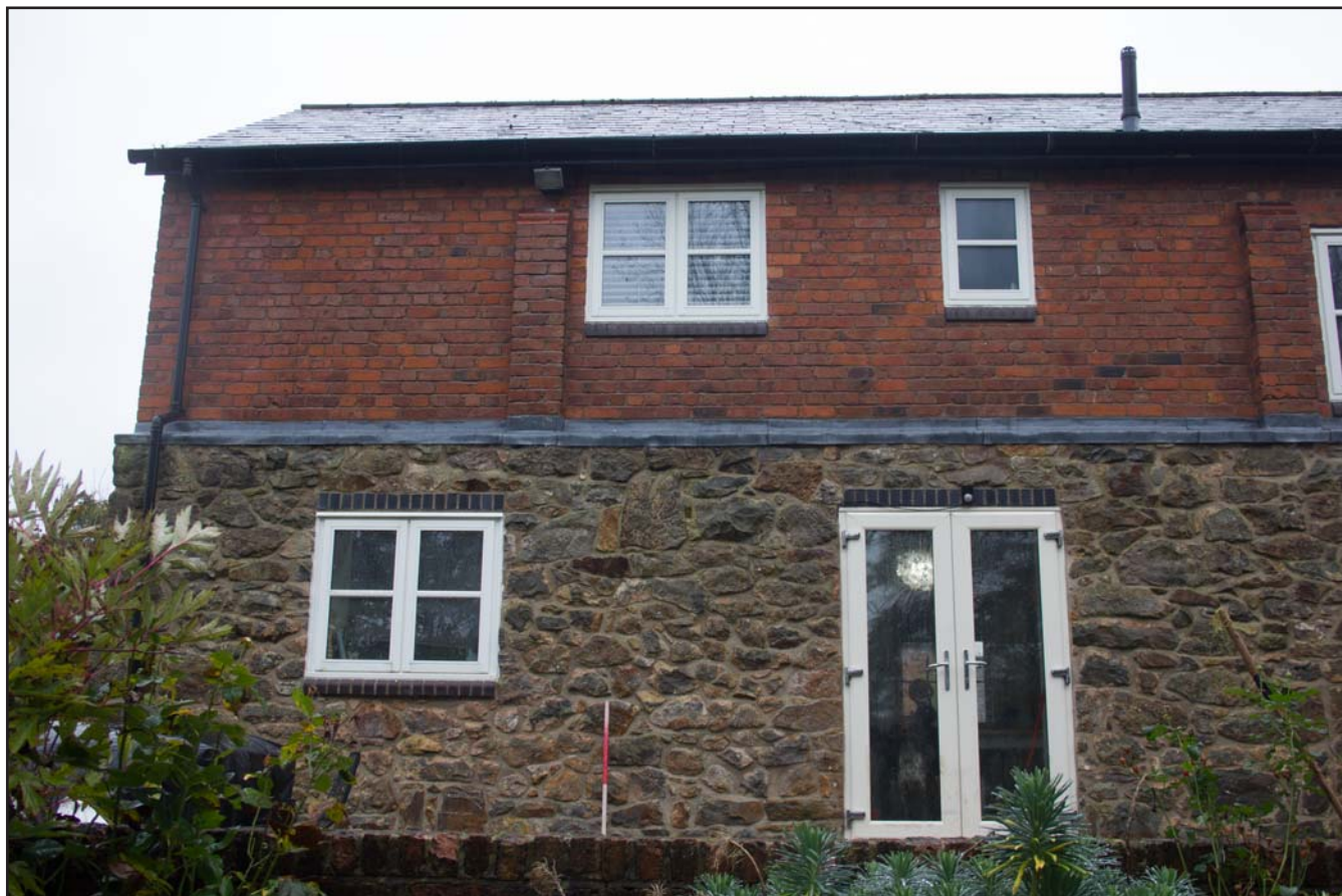
Plate 04: Left side of north western elevation of 5, Rackery Hall Mews, Rackery Lane, Llay, Wrexham - from the northwest - 1.00m scale
