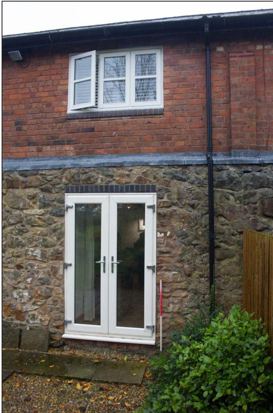
Plate 06: Right side of north western elevation of 5, Rackery Hall Mews, Rackery Lane, Llay, Wrexham - from the northwest - 1.00m scale
