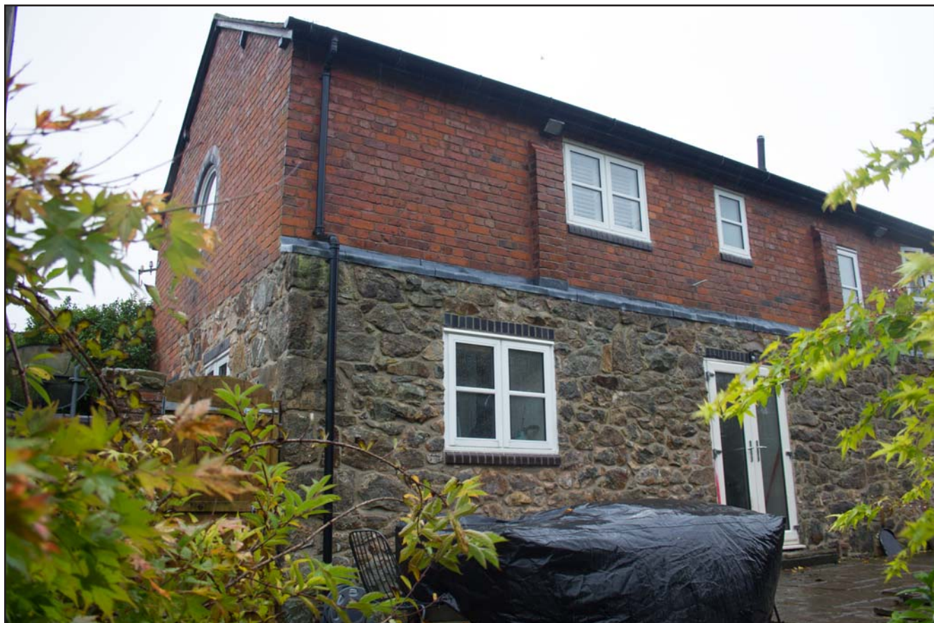
Plate 03: Oblique shot of north western and north eastern elevations of 5, Rackery Hall Mews, Rackery Lane, Llay, Wrexham - from the north - 1.00m scale
