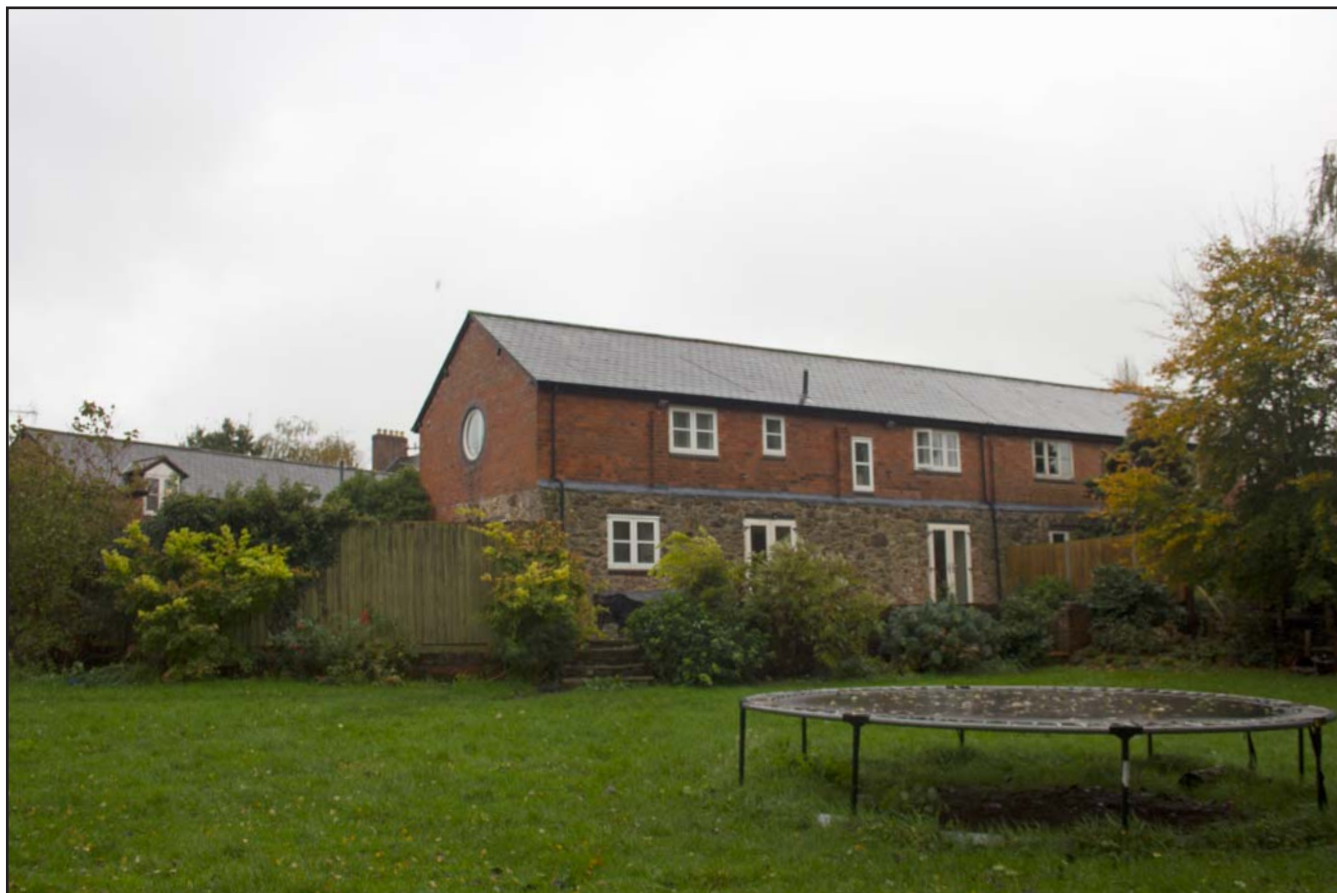
Plate 01: Long angle shot of north western and north eastern elevations of 5, Rackery Hall Mews, Rackery Lane, Llay, Wrexham - from the north - no scale
