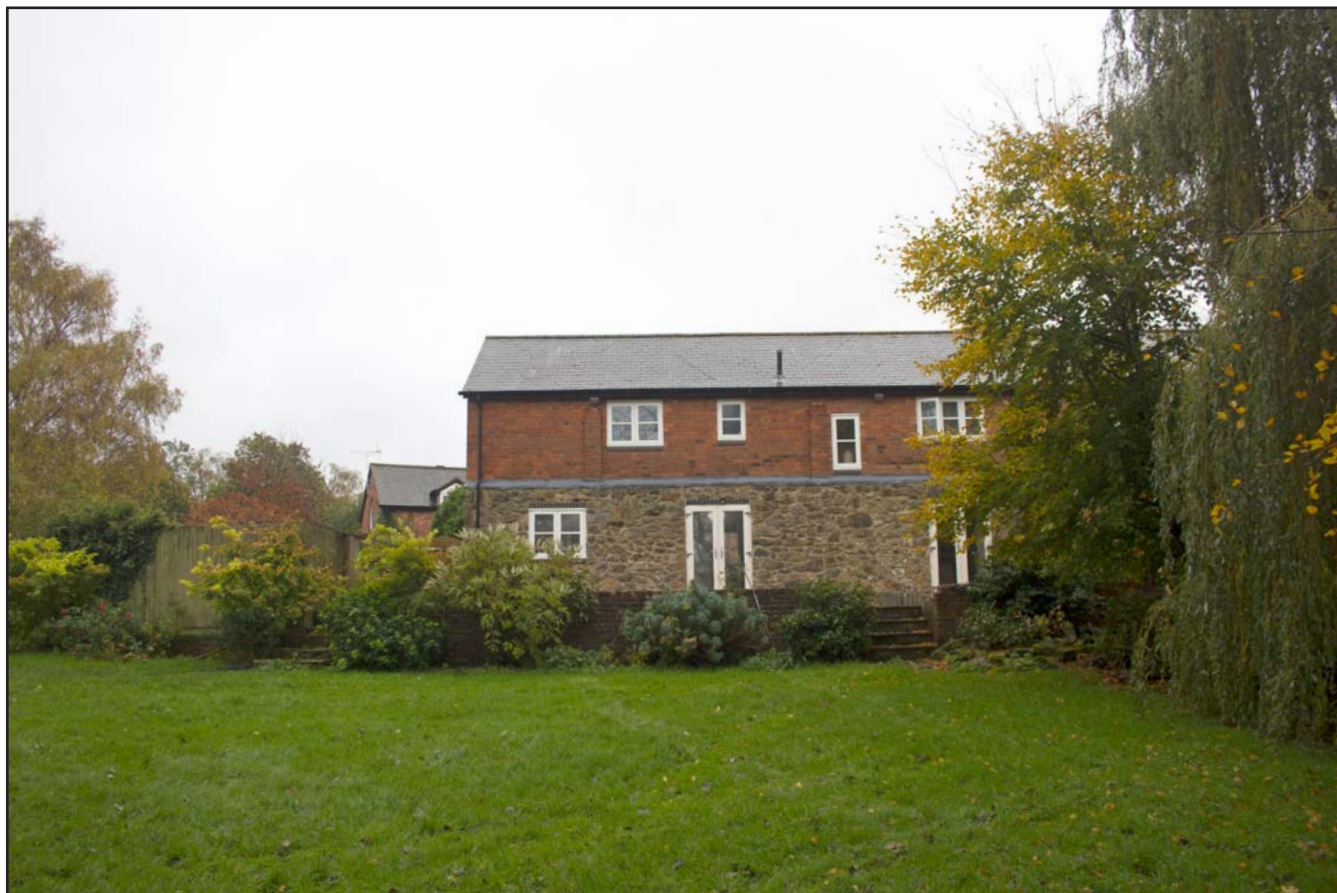
Plate 02: Long angle shot of north western elevation of 5, Rackery Hall Mews, Rackery Lane, Llay, Wrexham - from the northwest - no scale
