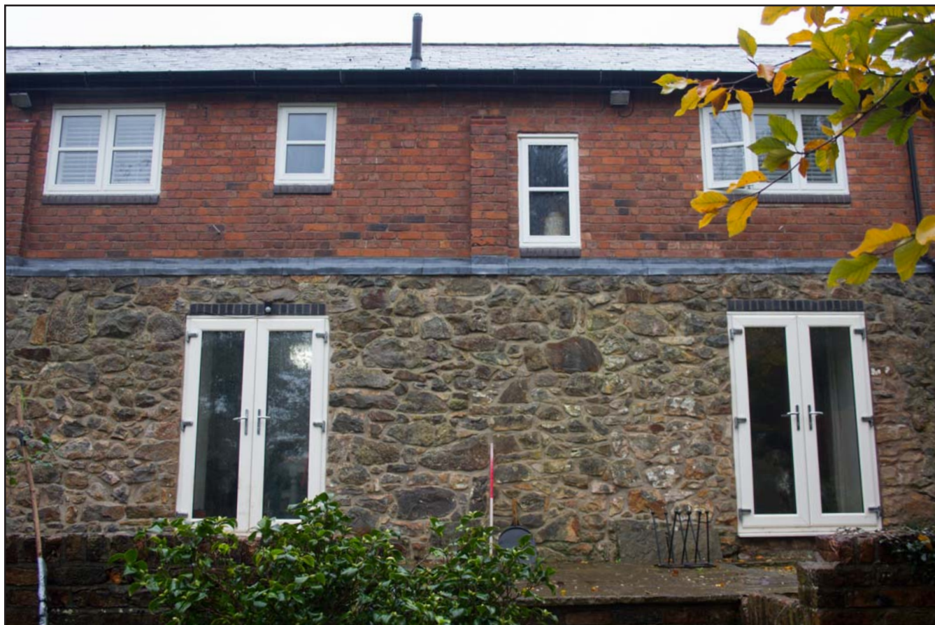
Plate 05: Centre of north western elevation of 5, Rackery Hall Mews, Rackery Lane, Llay, Wrexham - from the northwest - 1.00m scale
