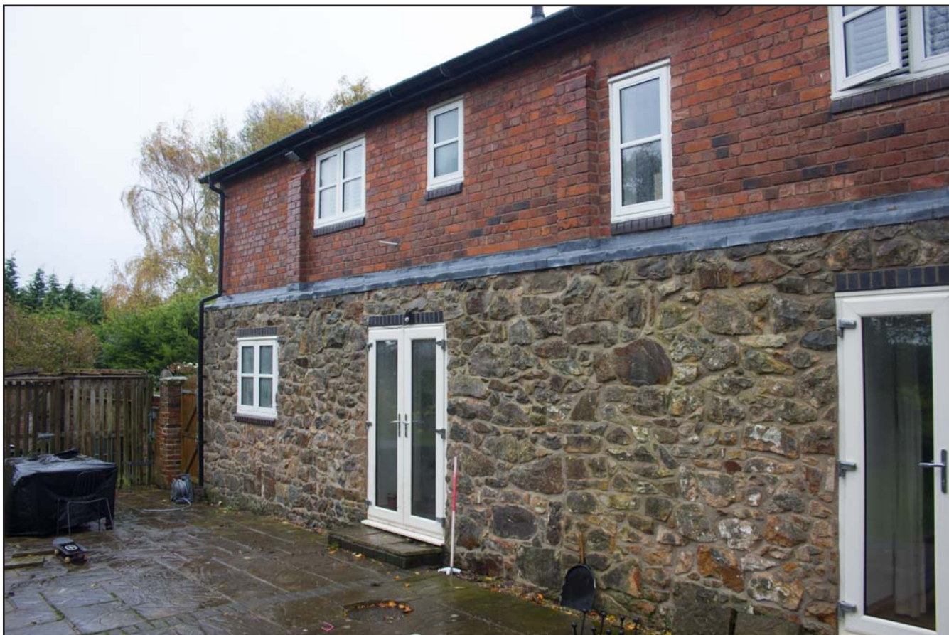
Plate 07: Oblique shot of north western elevation of 5, Rackery Hall Mews, Rackery Lane, Llay, Wrexham -from the west - 1.00m scale
