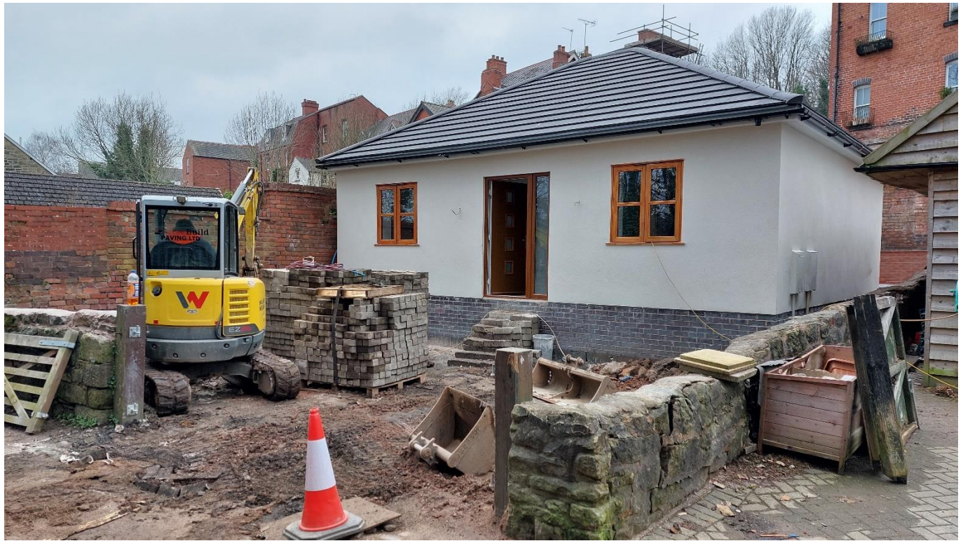
TP1 machine excavation
